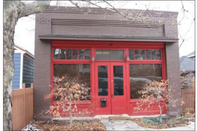
A good example of a one-part commercial block is the building at 361 N Main Street (ca. 1919).
