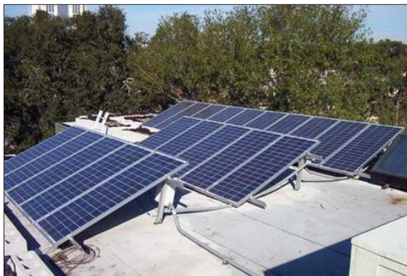
Rooftops may be an appropriate location for solar panels.
