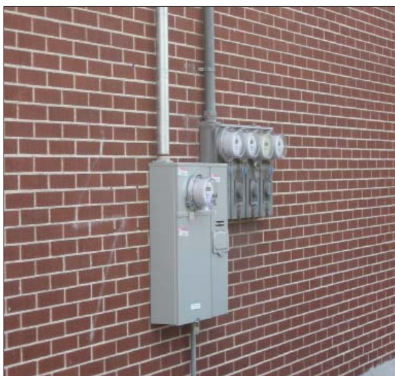
Meters are correctly placed on a secondary facade.
