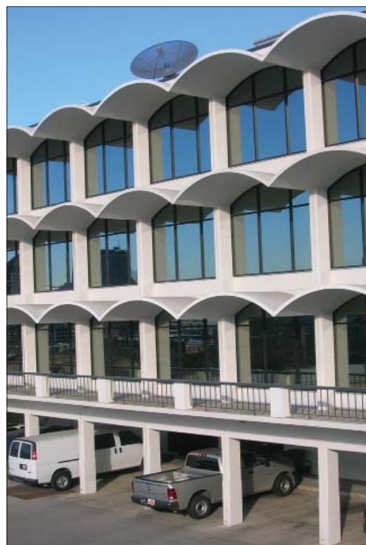
This satellite dish is appropriately placed towards the rear of the building.
