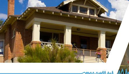
Unreinforced masonry buildings (URMs) were commonly built throughout Utah until the 1970s. Salt Lake City alone has more than 30,000 residential URMs. Seismic experts say those structures are among the most vulnerable types of buildings and are not likely to withstand the impact of any significant tremor.
