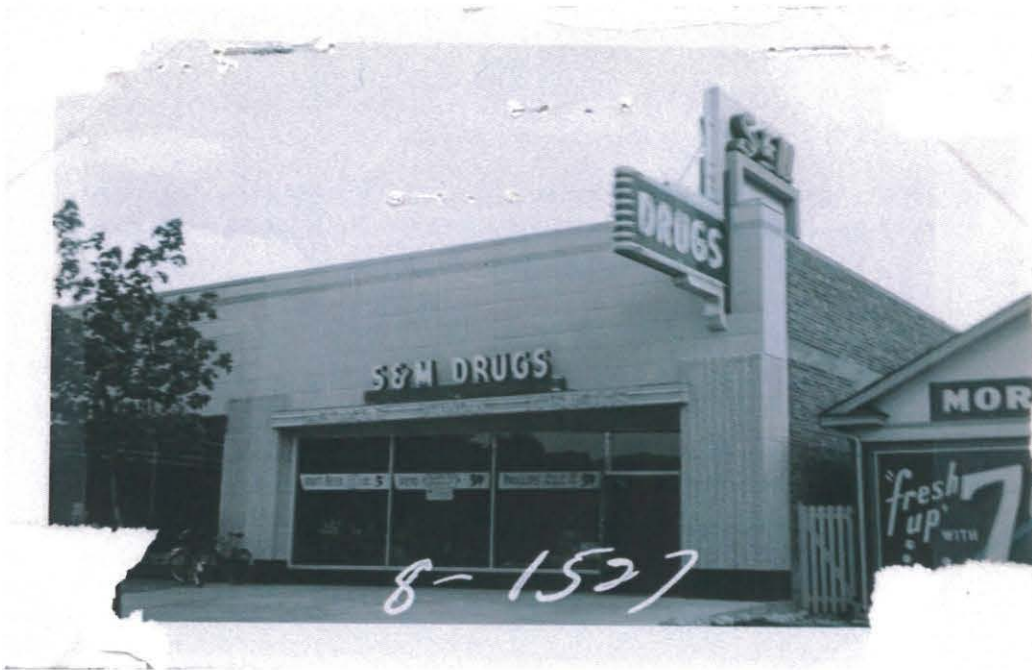
Historic Photo - 416 E 900 S – West End
