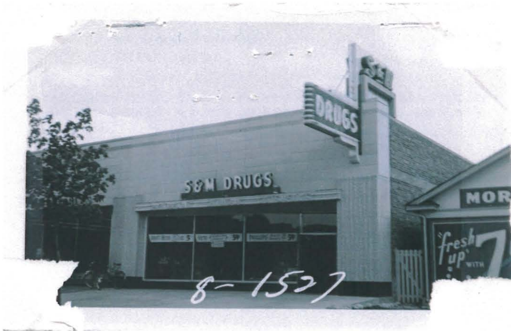
Historic Photo - 416 E 900 S – West End
