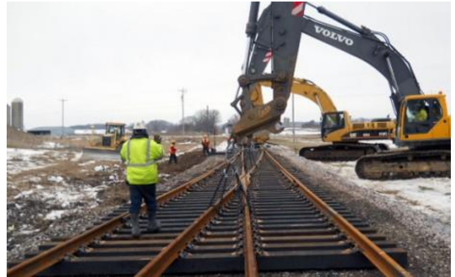
Source: Holubar Construction
