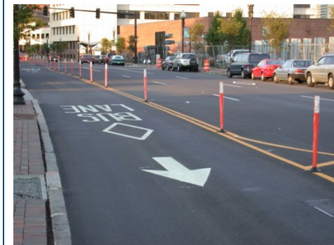
Contraflow bus lane in Boston, MA.
