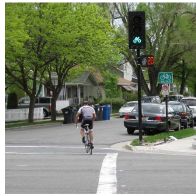
Bicycle signal treatment along 600 E neighborhood byway.
