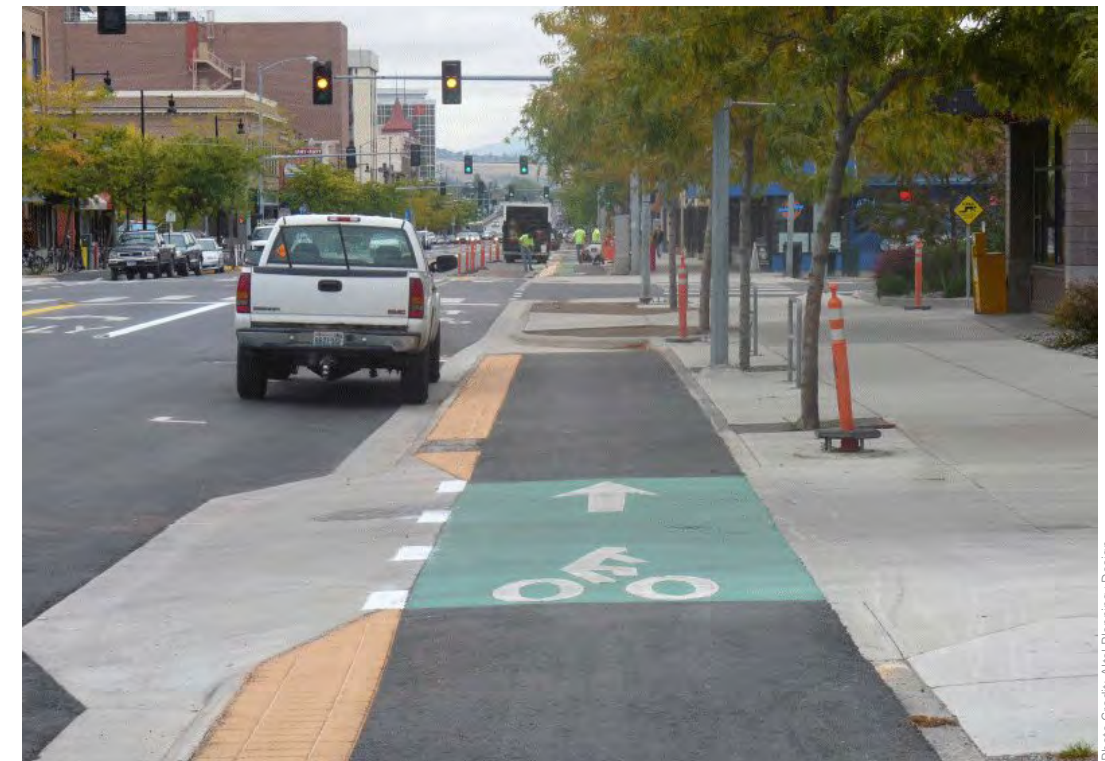
An example of a cycle track that is at the level of the sidewalk. This technique provides additional safety for cyclists to avoid conflicts with vehicles. The paving material is different from the sidewalk to signal the presence of the track to pedestrians.
