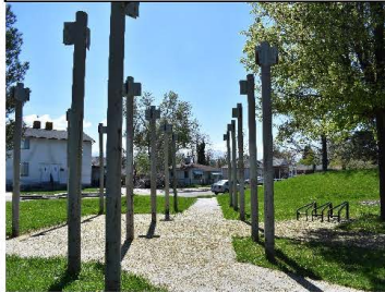
Failing Shade Structure Jackson Park
