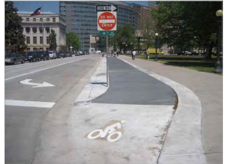
An example of a cycle track in downtown Denver. It is separated from the vehicle lanes by a curb and a change in grade. Photograph courtesy of Mike Lydon, The Street Plans Collaborative.
