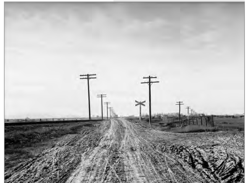
As late as 1918, there was very little in the way of development west of the tracks at 400 West. This photograph shows Indiana Avenue looking west. Photograph courtesy of the Utah State Historical Society.
