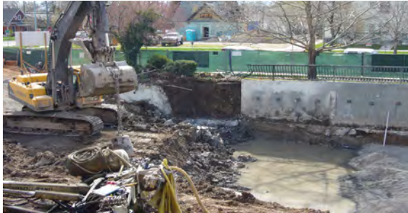
Ground water can have an impact on development. Often times, basements and subterranean parking structures are required to pump ground water to prevent it from damaging buildings.
