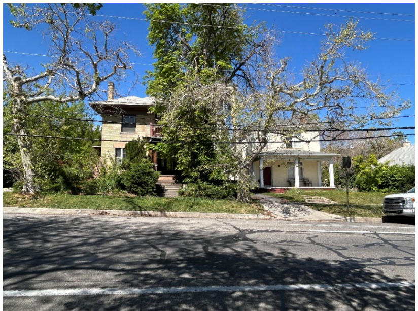
Nearby Residential Buildings
