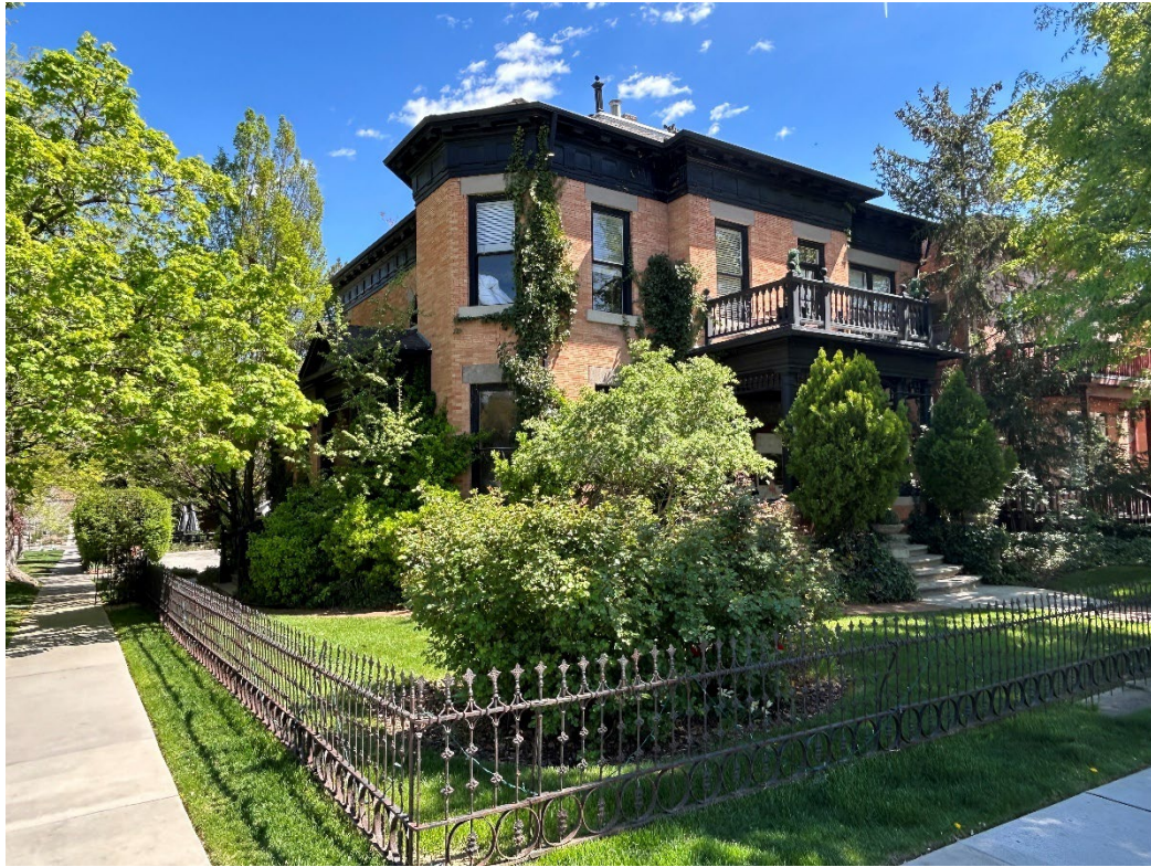
Ellerbeck Mansion from the corner of B St and 3 rd Ave
