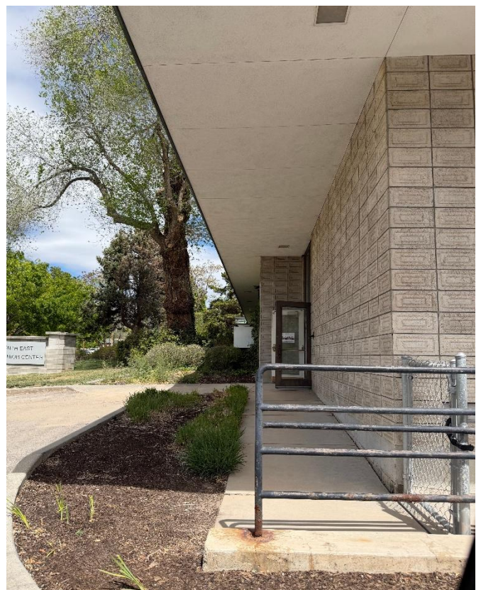
View of property from South Side exit ramp
