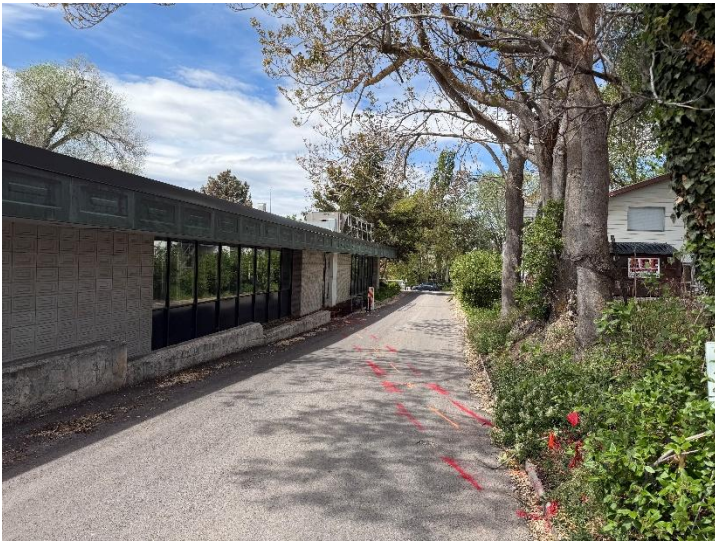
Entry ramp on North Side of property
