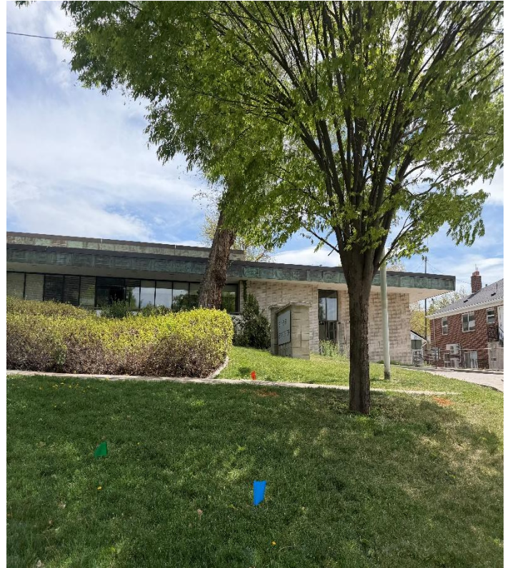
View of subject property from 1000 East
