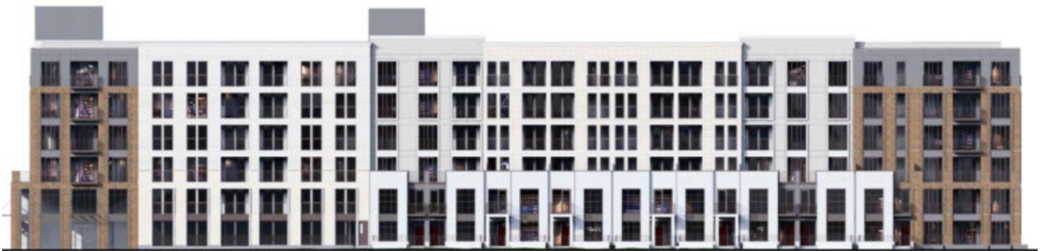
200 N Elevation – PD request is for 3'9" of additional building height, which allows the townhomes on 200 N to be elevated from the public sidewalk, creating a sense of privacy and security
