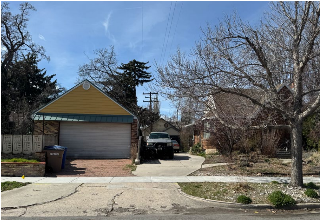
View looking West – 2554 S. Dearborn St. on the right of the photo. The accessory structure on the left and the garage behind the vehicles are all impeding on the alleyway that comes through from the West (2553 S. Chadwick St.)
