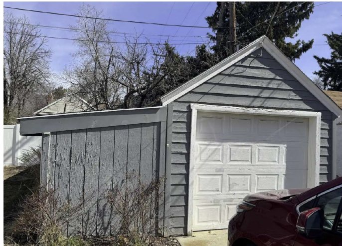
Existing garage -most likely built in the mid-1950s.
