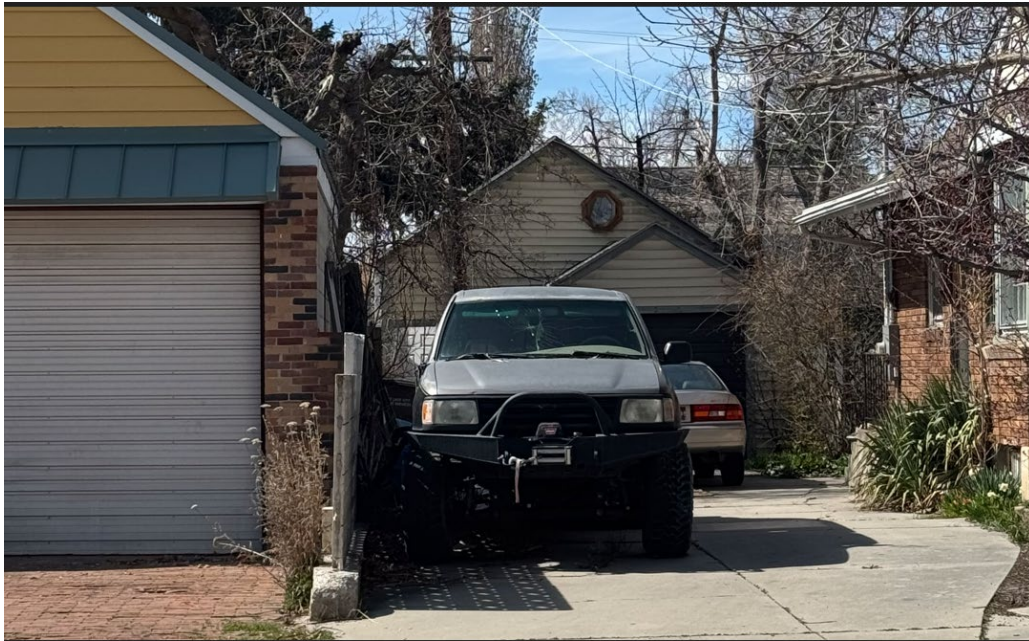
View looking West – close up of accessory structure and garage impeding on alleyway
