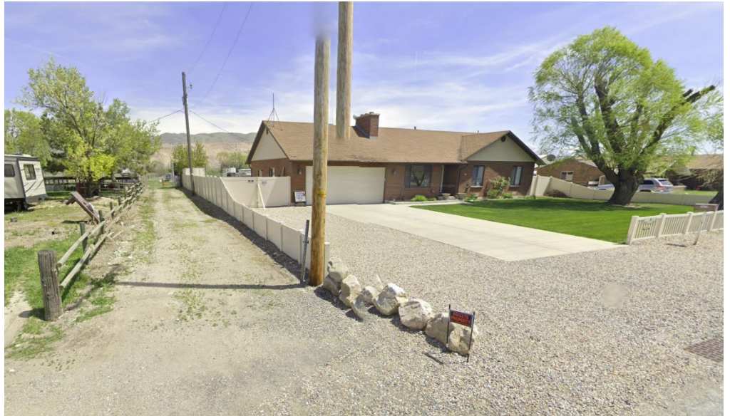
Existing home at 2620 N 2200 W
