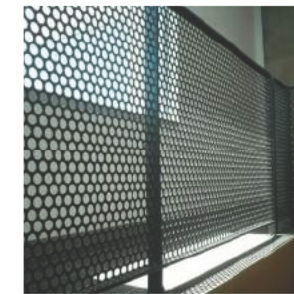
5. PERFORATED METAL PANEL RAILING
