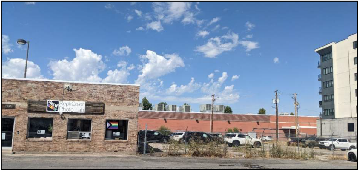
Subject Property (Building on Left to be Demolished)
