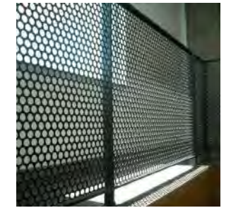
5. PERFORATED METAL PANEL RAILING
