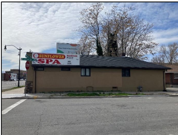
Commercial building to the north
