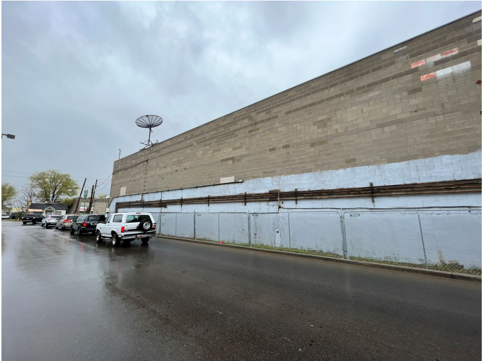
View of existing west building from Costco driveway
