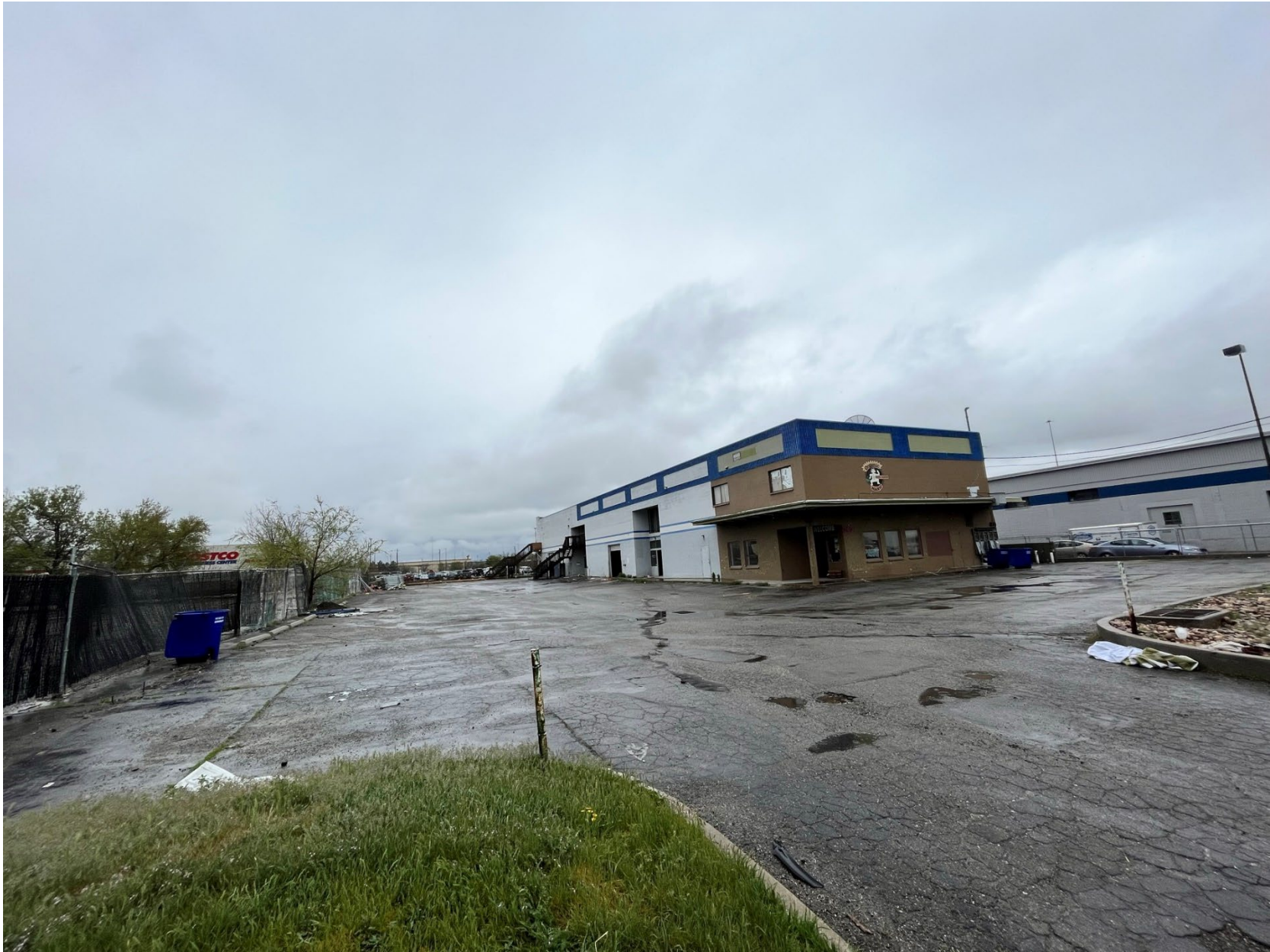
Existing west building on subject property (old wellness store and restaurant)
