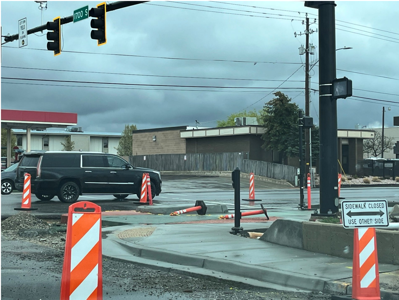
Construction on 300 West with new bike lane and sidewalk
