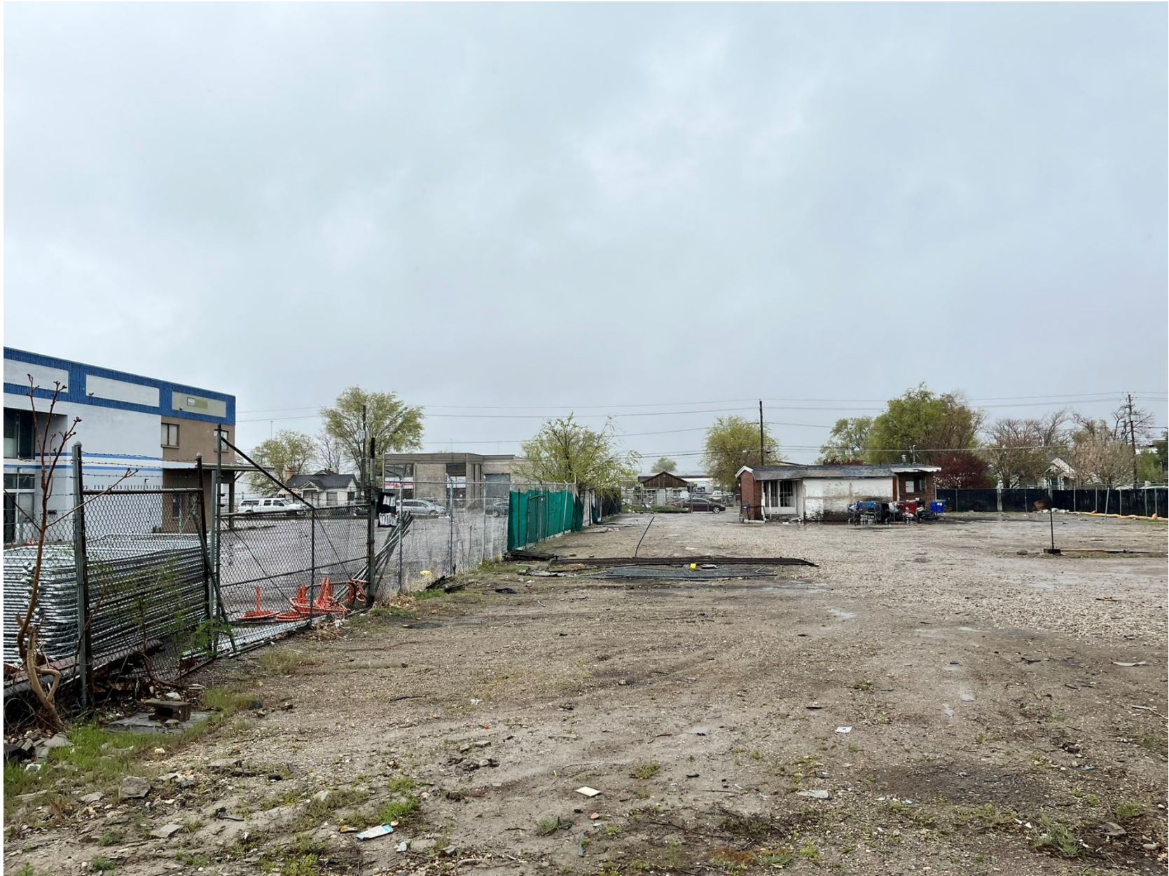
Existing fence on property to be removed
