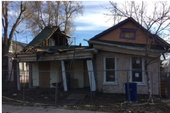
Figure 5 – Contributing house in the Avenues Local Historic District was severely damaged in 2017 after interior demolition resulted in the destabilization of the structure.
