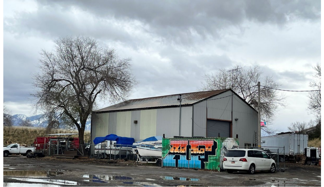
1007 South 500 West, facing southeast
