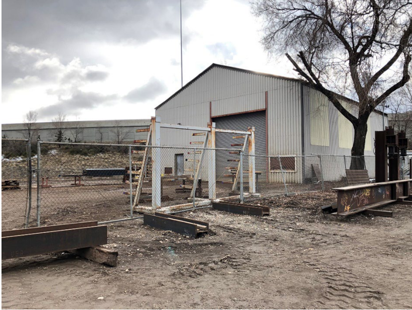
1007 South 500 West, facing southwest
