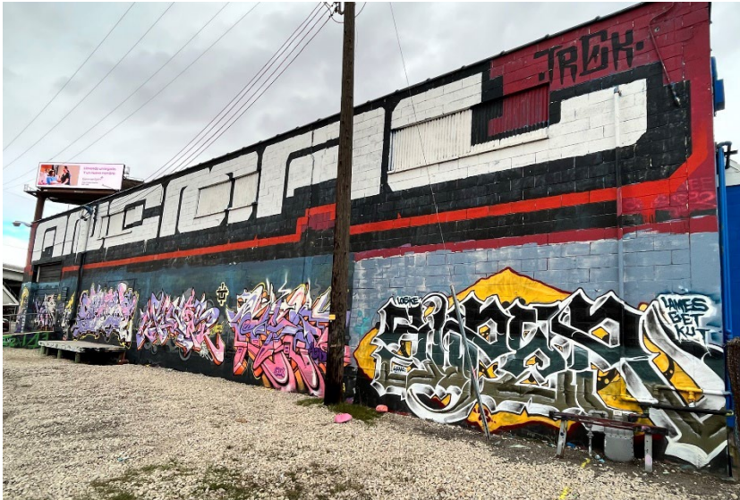
South wall of 1005 West 500 South
