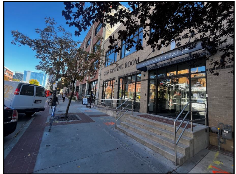
Public Entrance Looking East
