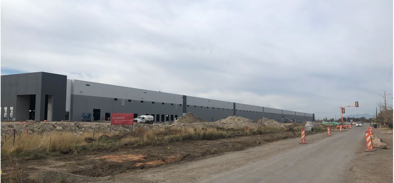
View from the south looking northwest along 2200 West. – application properties ahead on the right
