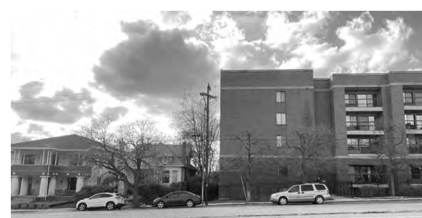
680 E 100 S LOCAL + NATIONAL CENTRAL CITY HISTORIC DISTRICT YEAR BUILT: 1987 4 STORY
