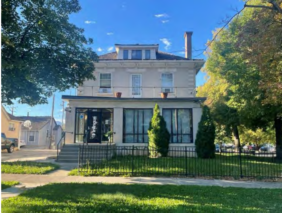
Existing structure at 602 E 300 S
