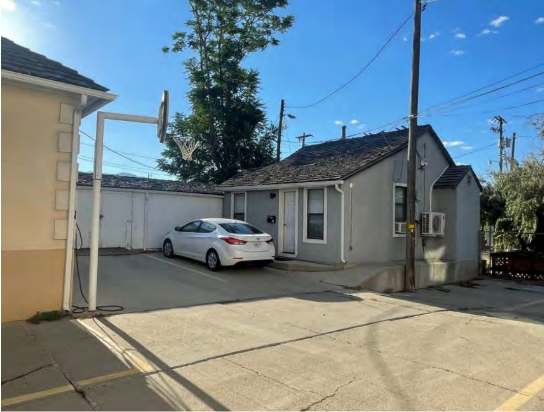
Existing structure at 614 E 300 S
