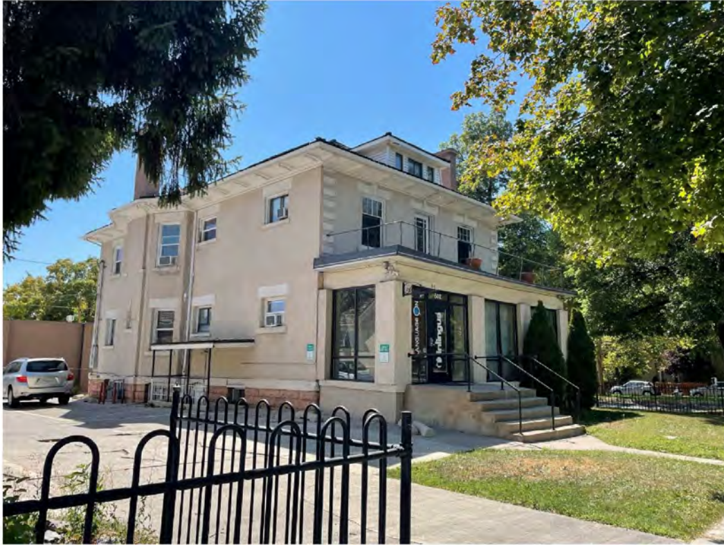
Front/North and Side/East Elevations
