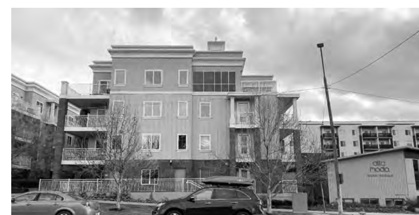
556 E 300 S LOCAL + NATIONAL CENTRAL CITY HISTORIC DISTRICT YEAR BUILT: 20121 4 STORY
