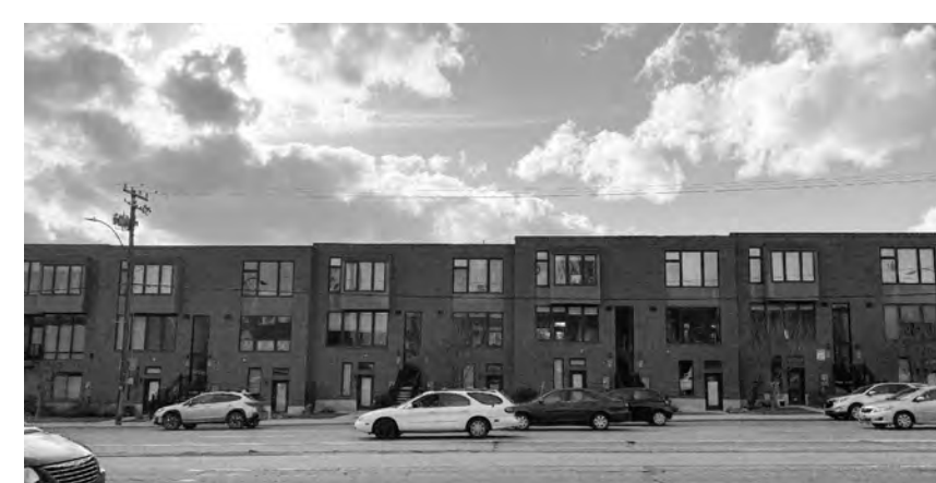
676 E MARKEA AVE LOCAL + NATIONAL CENTRAL CITY HISTORIC DISTRICT YEAR BUILT: 2011 3 STORY
