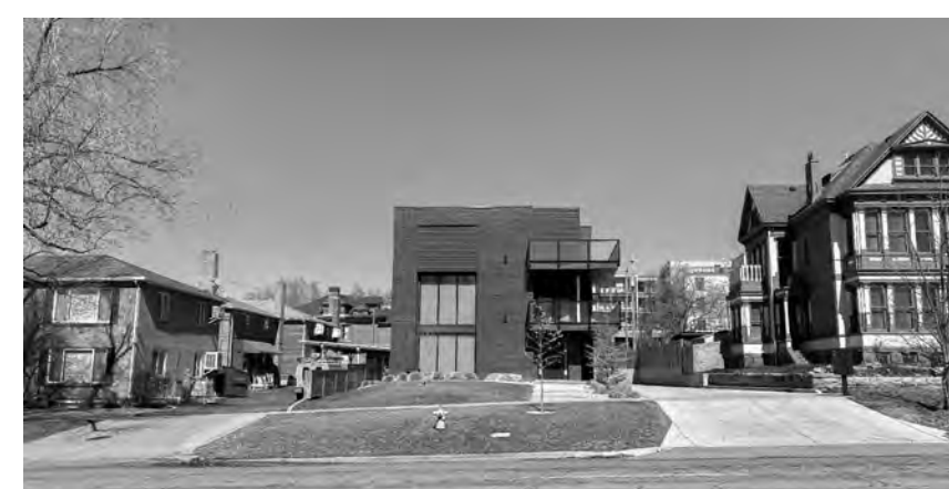
611 E 100 S LOCAL + NATIONAL CENTRAL CITY HISTORIC DISTRICT YEAR BUILT: 2018 3 STORY
