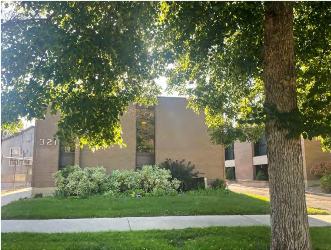
Existing structure at 321 S 600 E
