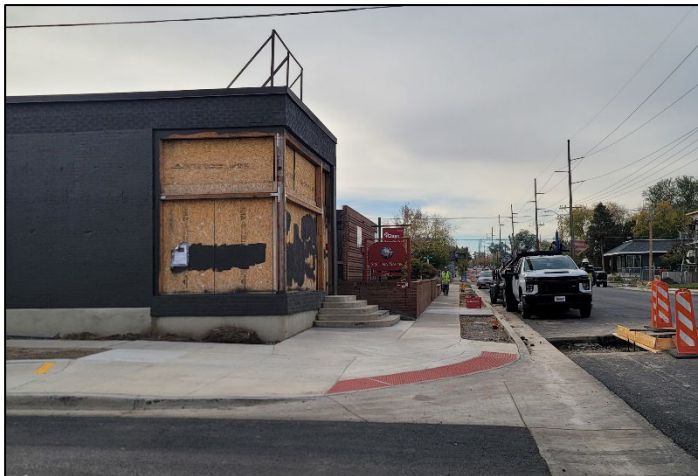
View of north & front facade, looking down 1100 E
