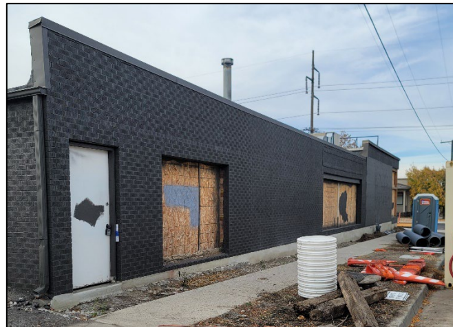
Northern facade of building
