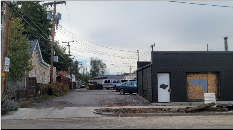
View of east facade of building and alley
