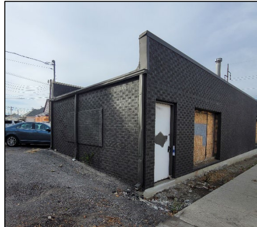
East facade of building
