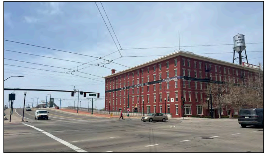
VIEW OF HARDWARE OFFICE FROM NORTH TEMPLE AND 400 WEST
