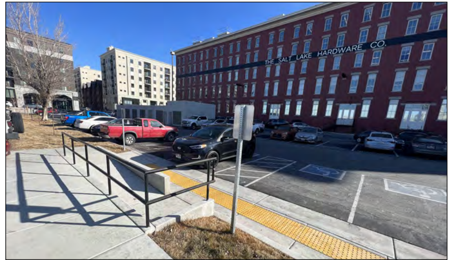
VIEW TO EAST
