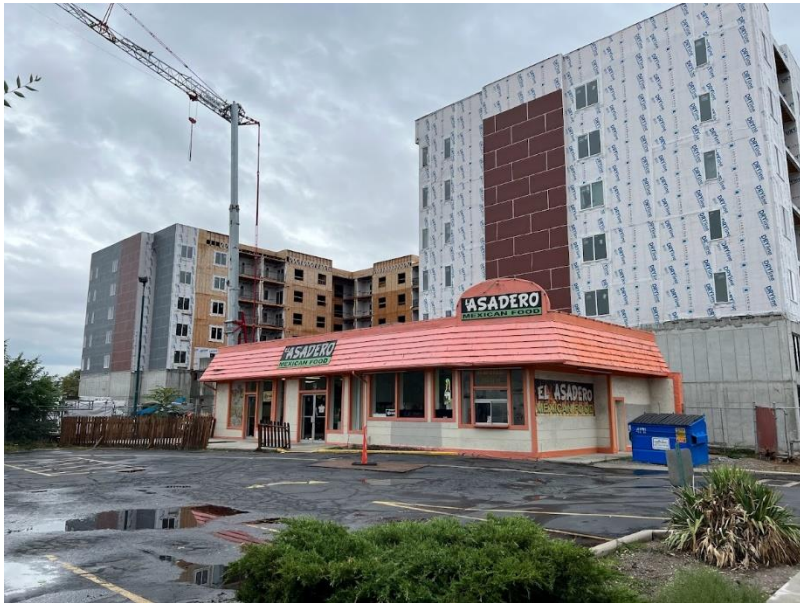
Project site looking southwest toward Building A
