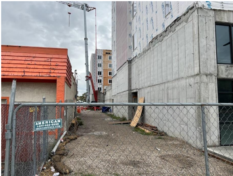
Alleyway between Building A and B
