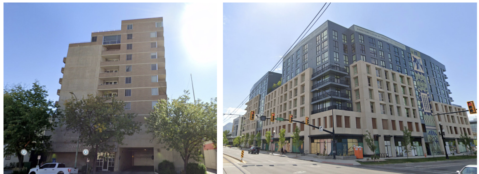
Figure 6- Broadway Tower (left) and Avia (right)
