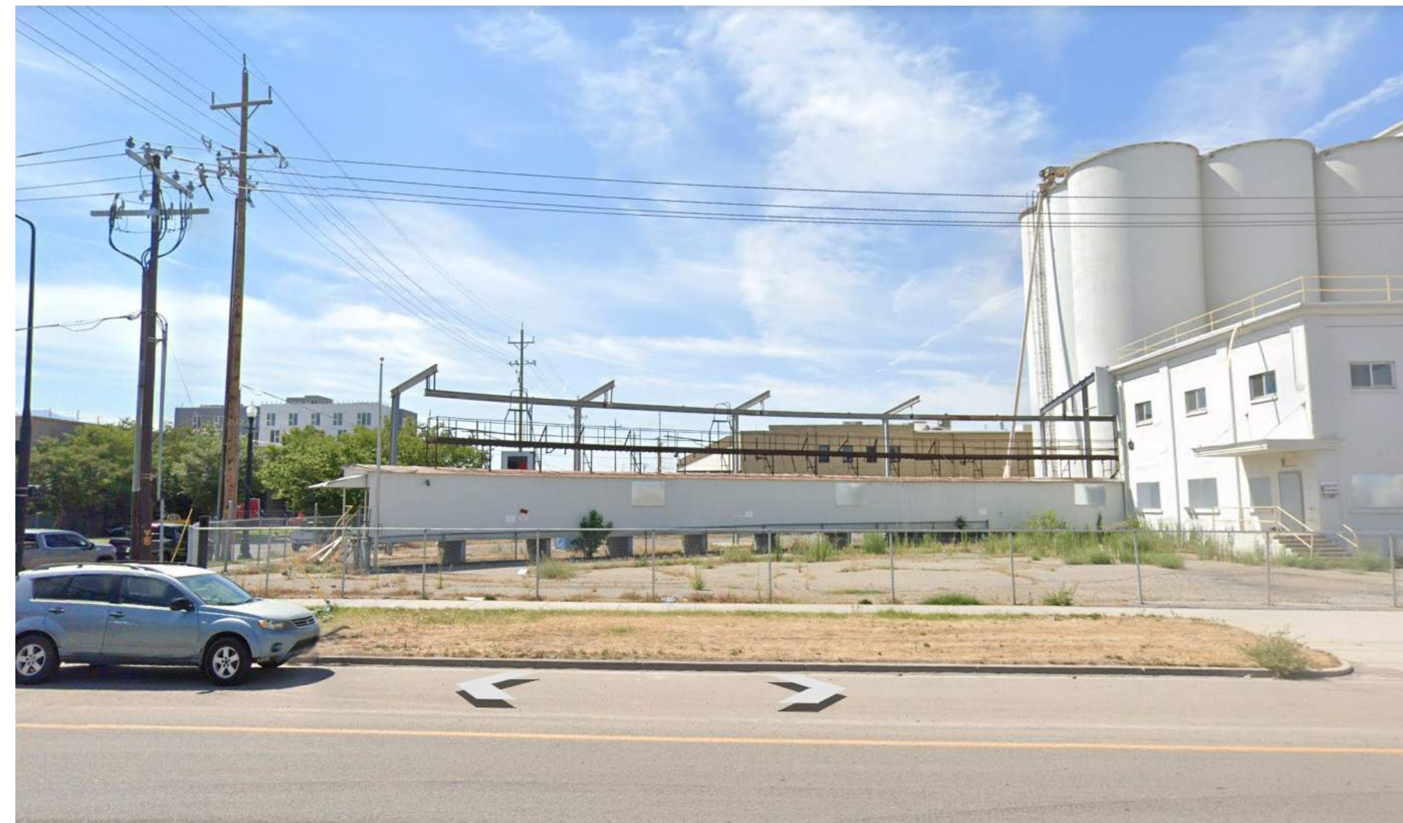
SILOS NORTH ELEVATION - EAST
