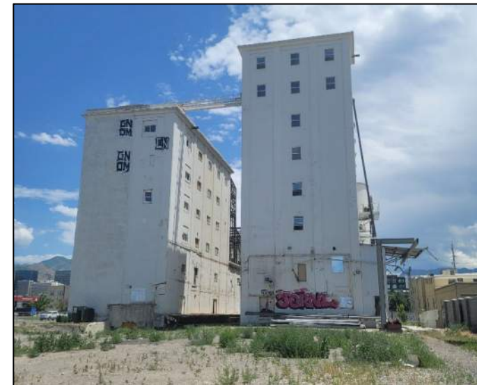
Central to the site - looking towards silos (east)
