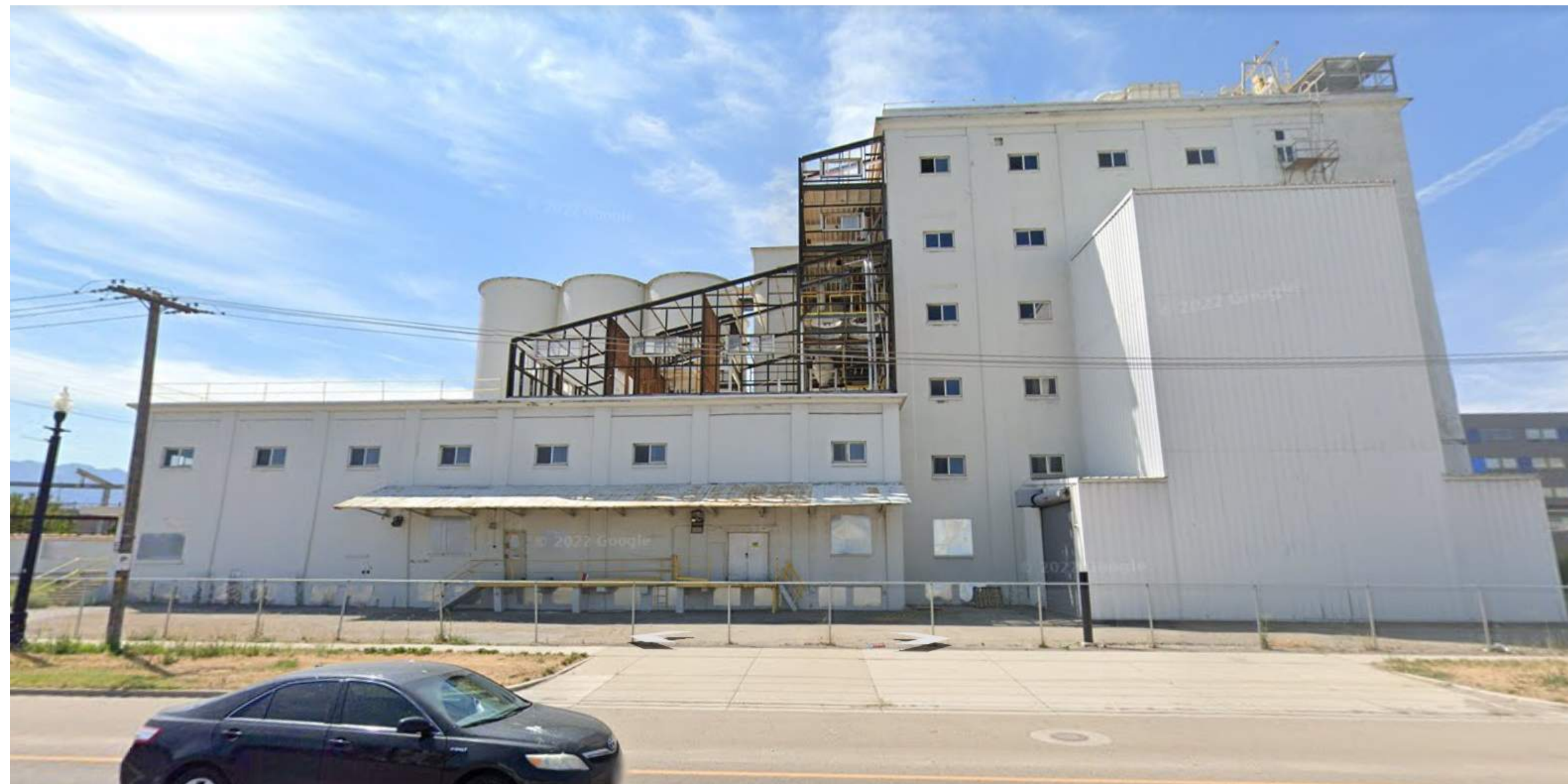
SILOS NORTH ELEVATION - WEST
