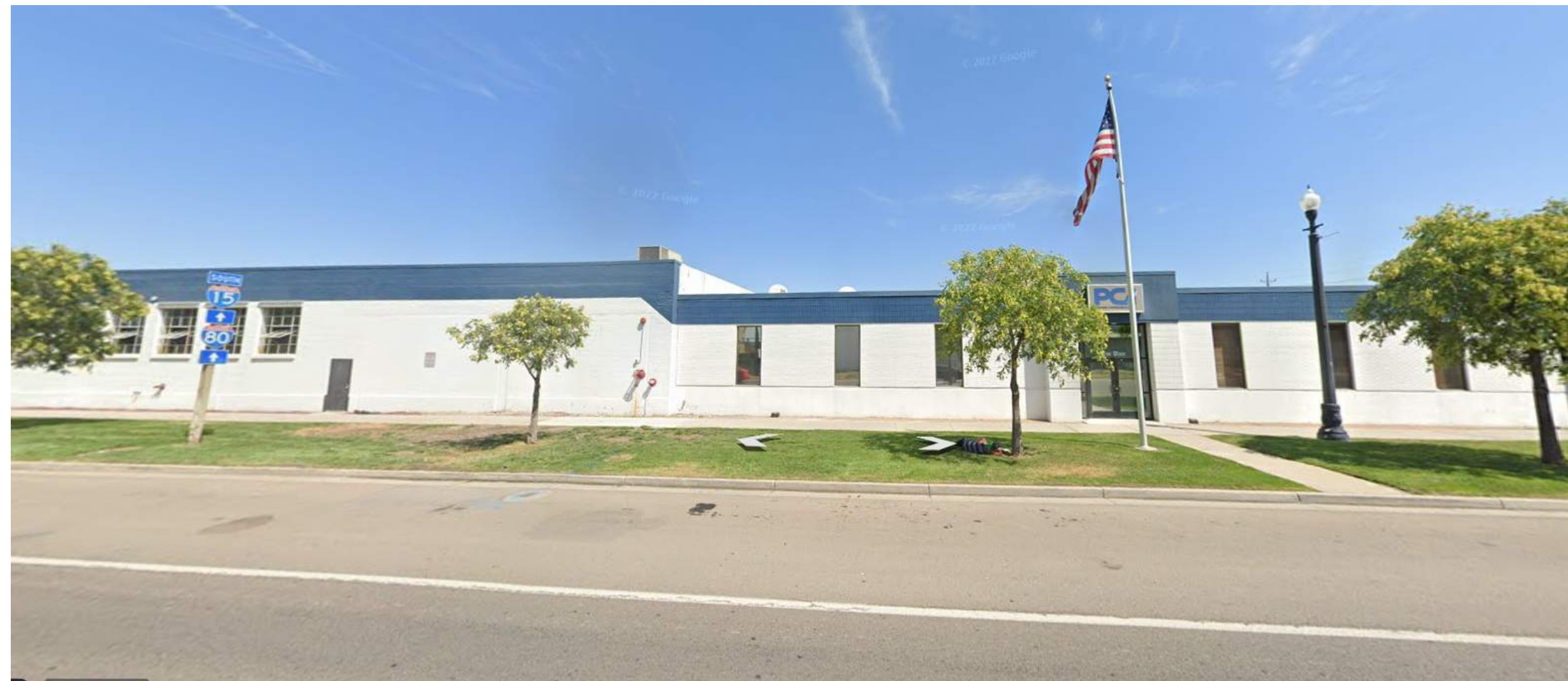
PACKING CORPORATION OF AMERICA SOUTH ELEVATION - EAST
