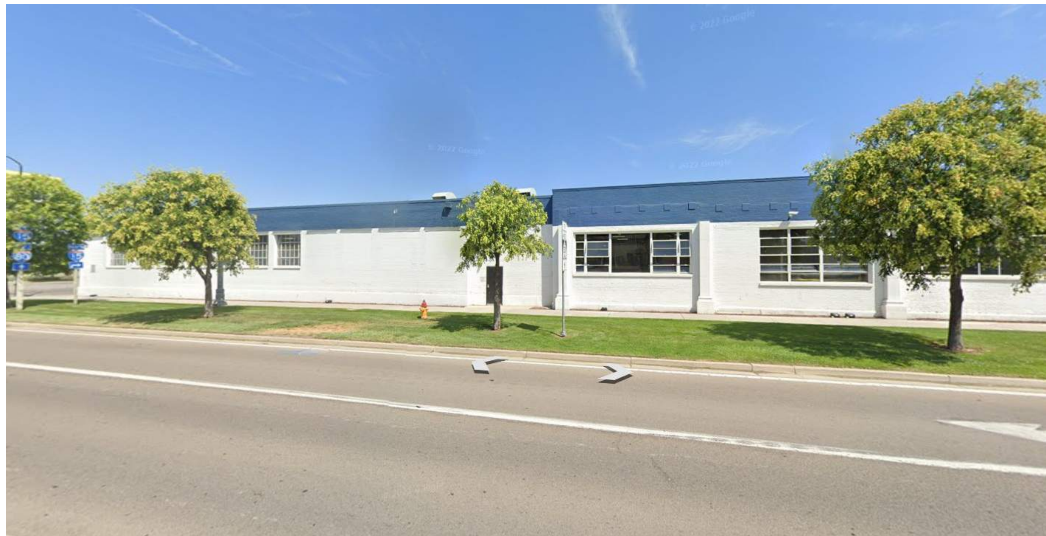
PACKING CORPORATION OF AMERICA SOUTH ELEVATION - WEST
