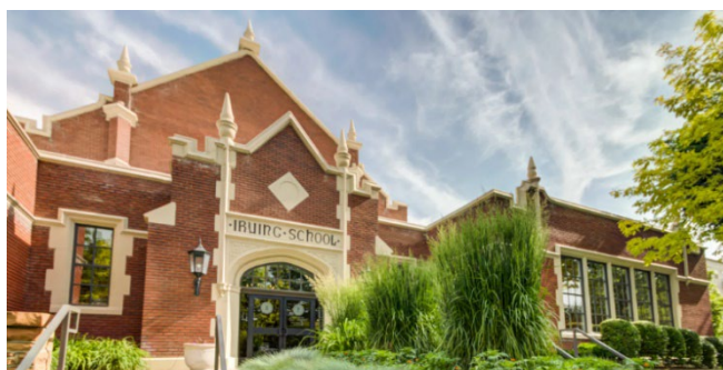
What was the Irving Junior High School constructed in the late 1920's, is now home to the Irving Schoolhouse Apartments and contains approximately 230 1- and 2-bedroom apartments.
