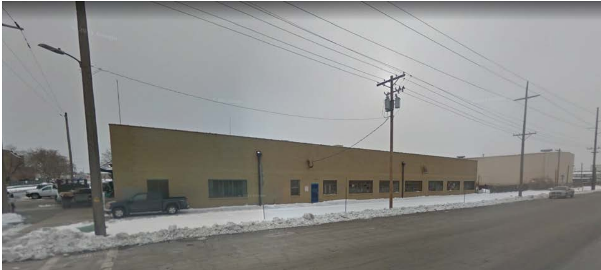
View of existing site from 700 South looking south. Note: existing power lines to remain.
