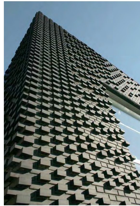
BRICK DETAILING - We are showing a brick pattern that wraps the corner on the ground level to bring the pedestrian's interest into the alley. To make a clear connection between the base and the middle of the building, the brick detail is simplified on the upper stories.
