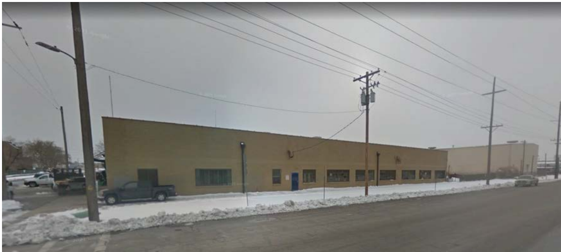
View of existing site from the corner of 400 West and 700 South.
