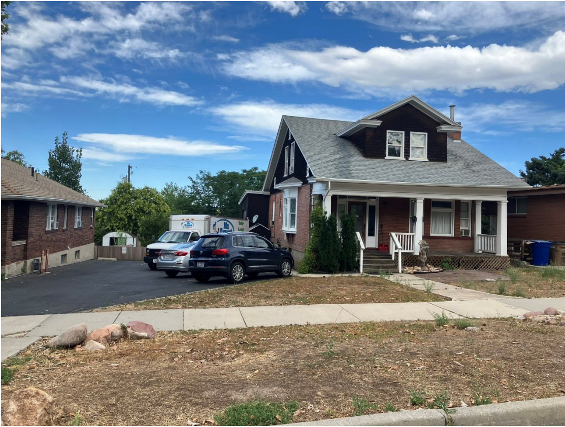
Existing triplex and parking area
