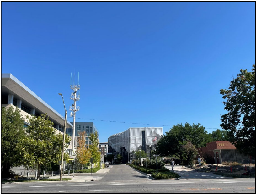
Public Safety Building, antennas, and westernmost building
