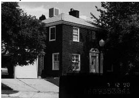
1425 E Laird Circle (A): 16-09-353-041 1939/35 Colonial Revival
