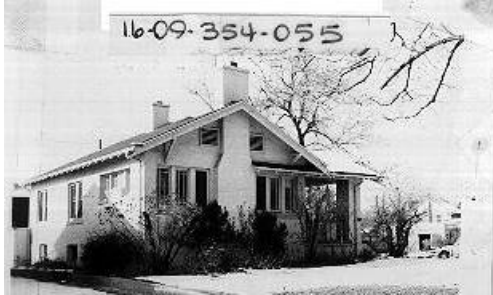
1480 E Laird Ave (B): 16-09-354-055 1923 Bungalow Original photo house side facing 1500 East
