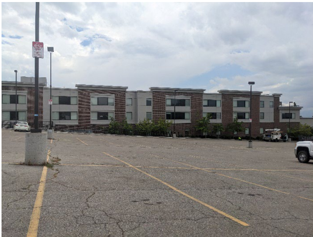
Commercial Development to Rear of Properties (South)
