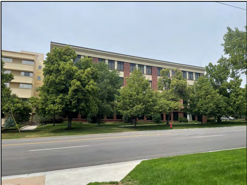
Property to the north: Holy Cross/Salt Lake Regional
