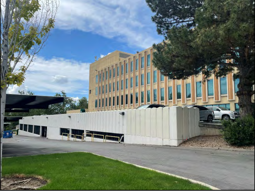
Subject property – Southeast corner
