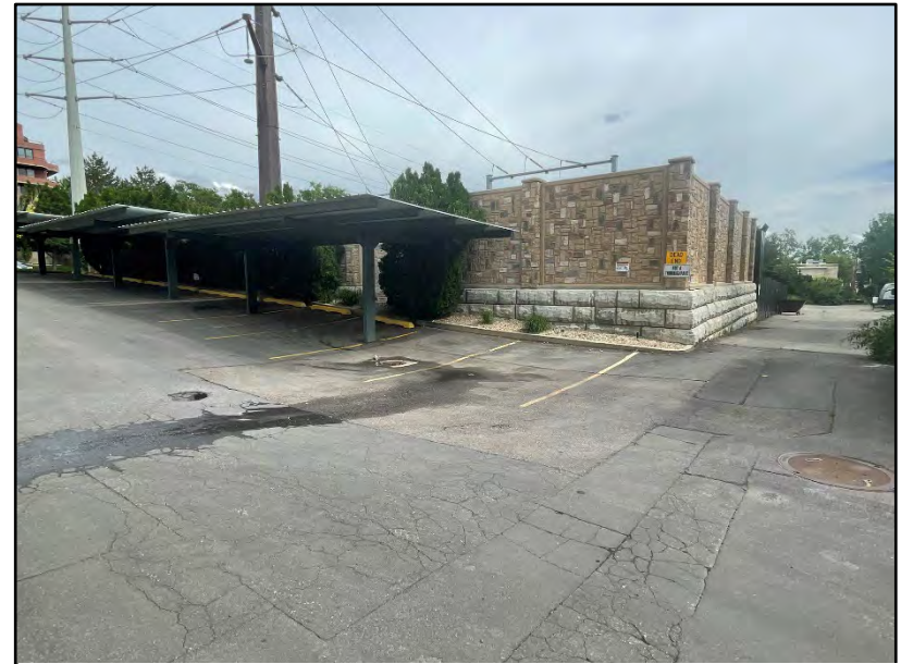
East-west alley, carports, and entrance to north-south alley
