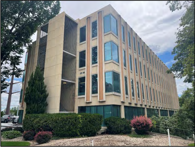
Subject property – Northeast corner
