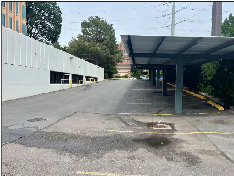
Subject property – Alley and carports (no changes proposed), facing east
