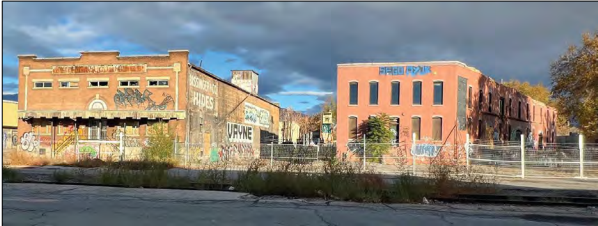
Existing Hide building (left) & Pickle building (right)
