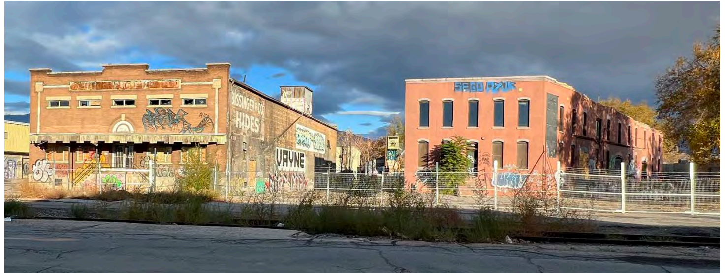
Existing Pickle and Hide buildings facing 400 West
