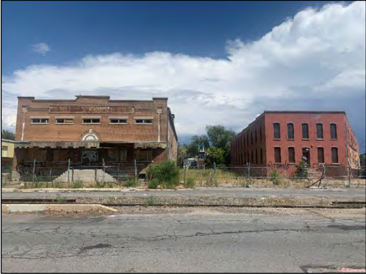
Historic Pickle & Hide structures & the front of the new development on 400 W
