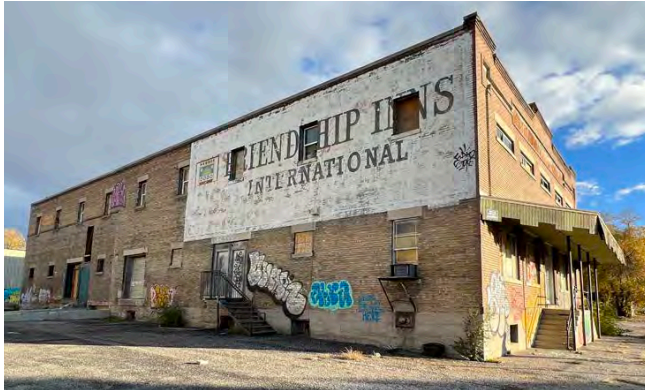
Northern facade of existing Hide building
