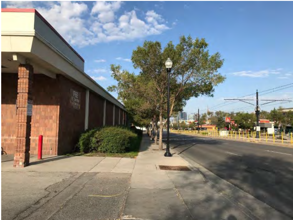
North façade of OfficeMax and 400 South, facing west
