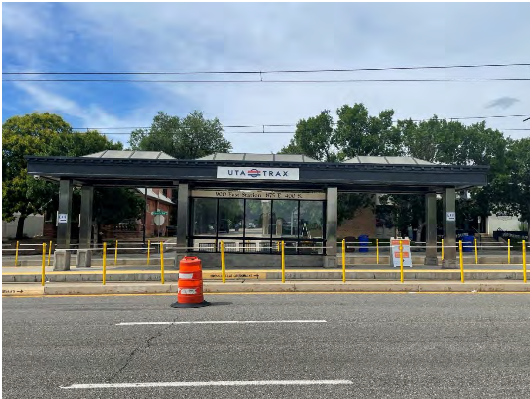
400 South, 900 East Trax Station to the north of the subject property
