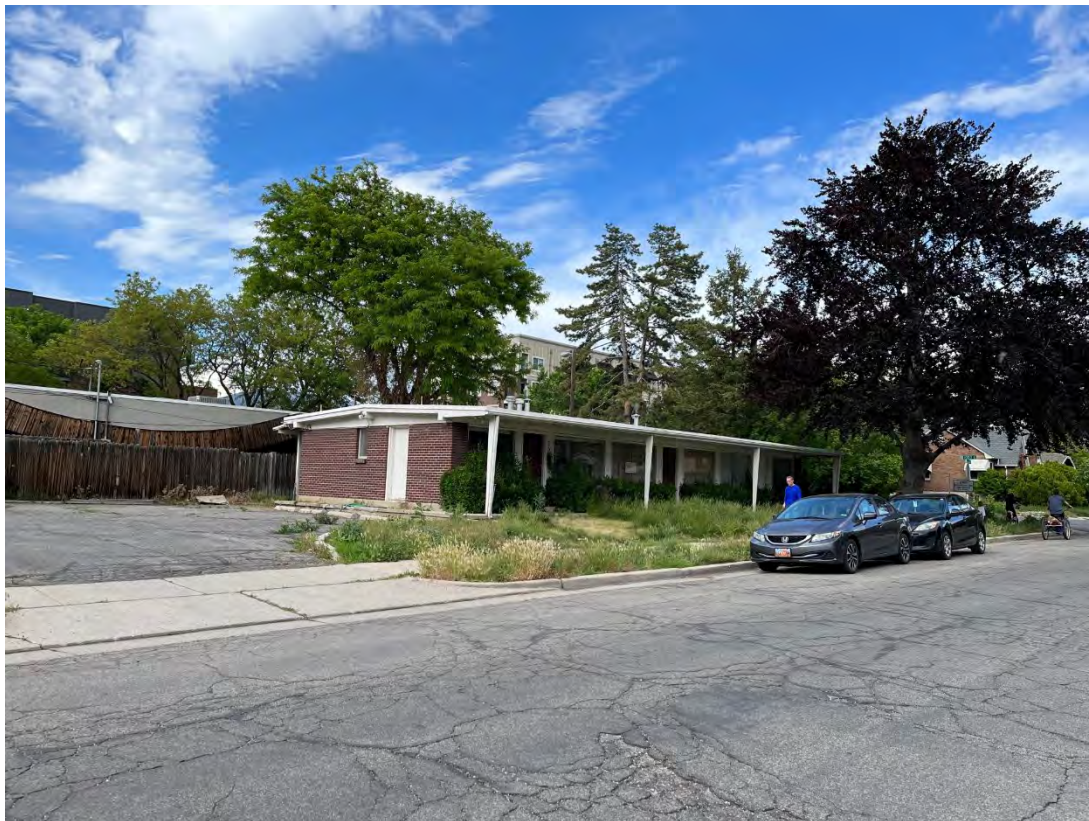
Office building to be demolished on Elm adjacent and to the east of the Victorian mansion.
