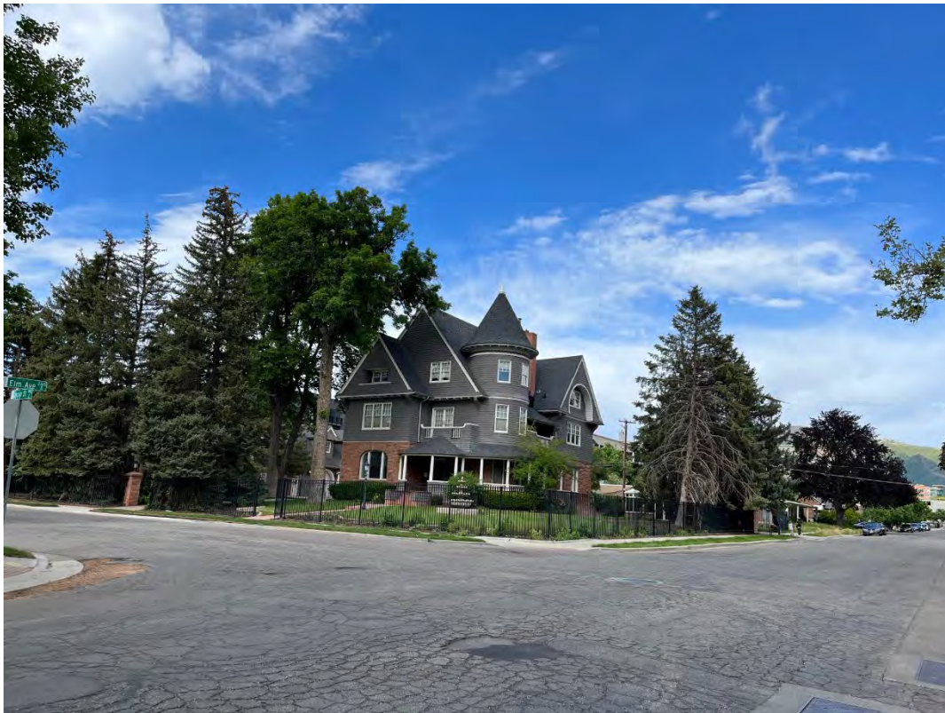
Victorian mansion on the corner of Lincoln and Elm to be preserved.
