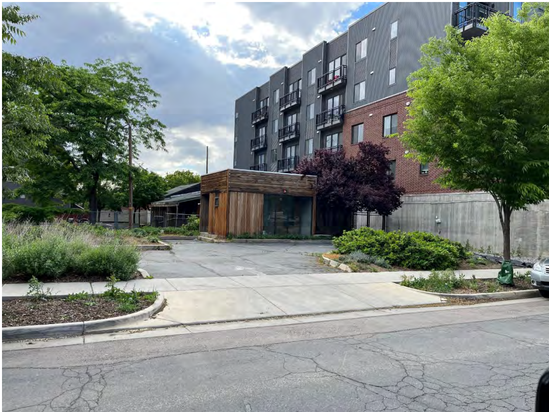
Building at 2134 S. 1000 East to be demolished.
