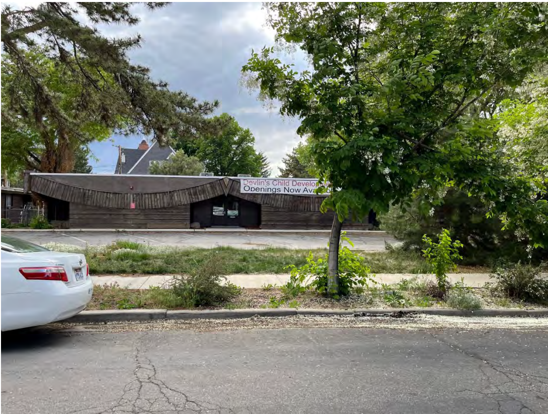
Building at 2156 S. 1000 East to be demolished.
