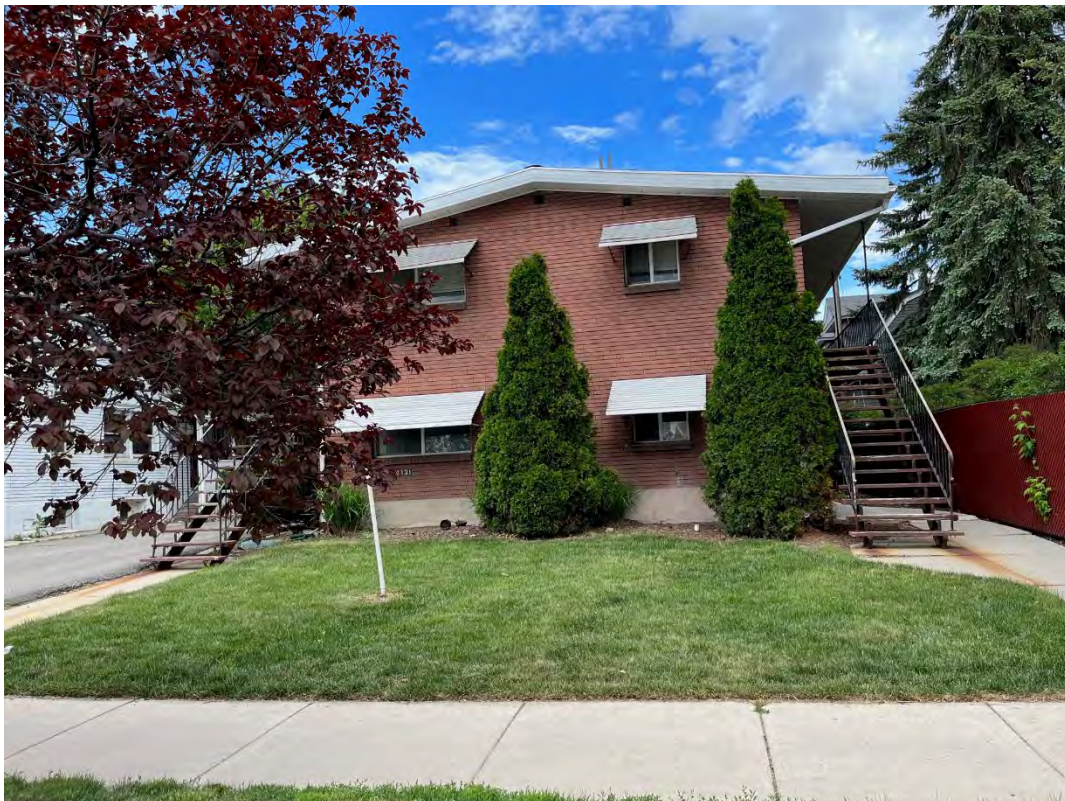
Apartment building at 2131 N. Lincoln St to be demolished.
