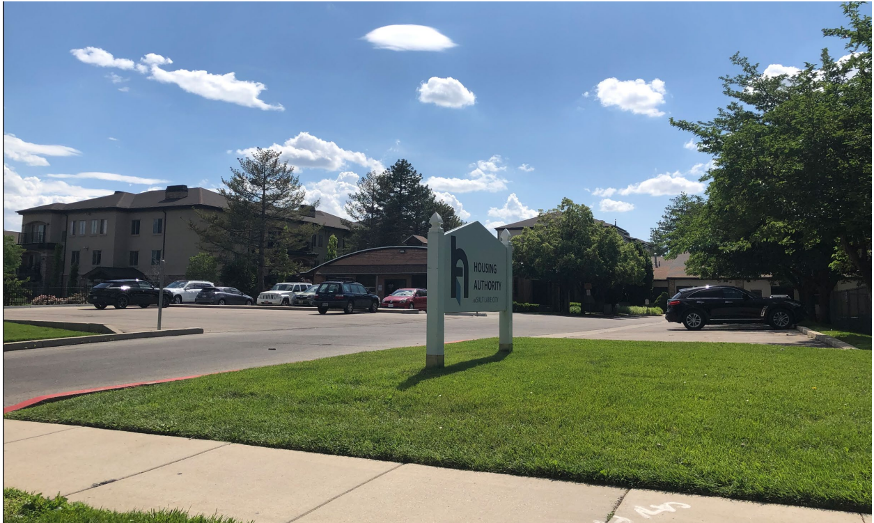
Housing Authority office building – down the street to the south.
