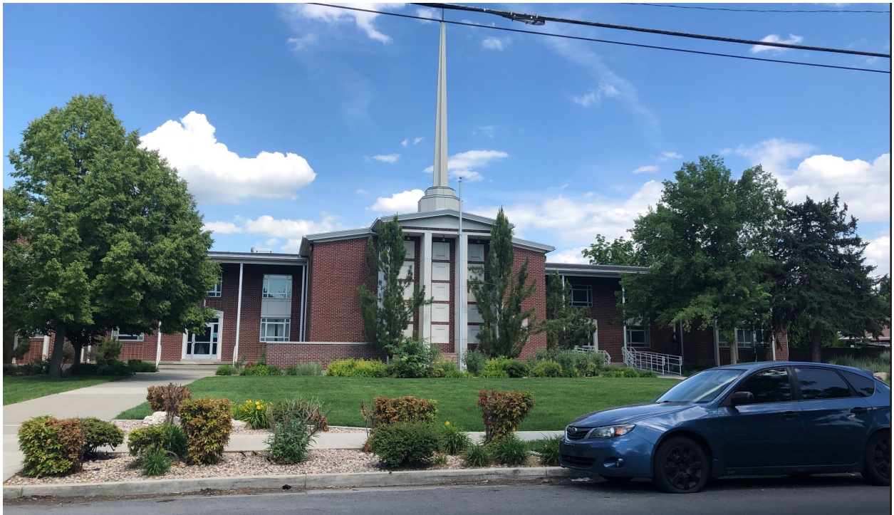
Church on the east side of West Temple to the south.
