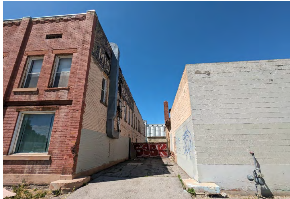
Proposed location of a midblock walkway, looking north from 600 S.
