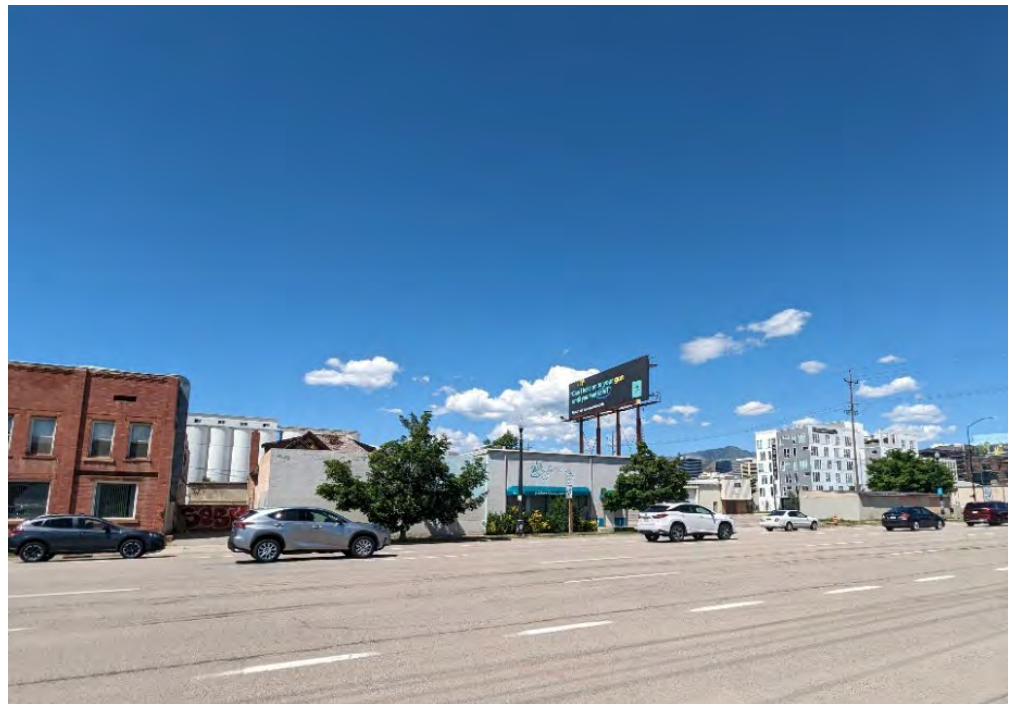
Proposed site of Building 2 along 600 S
