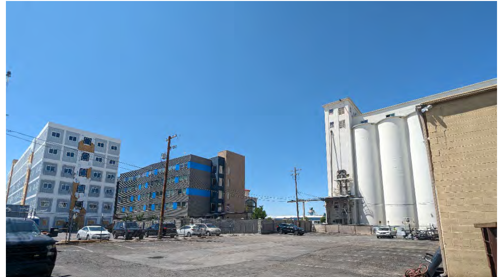
Proposed site of Building 1, southeast corner at the intersection of the midblock walkways
