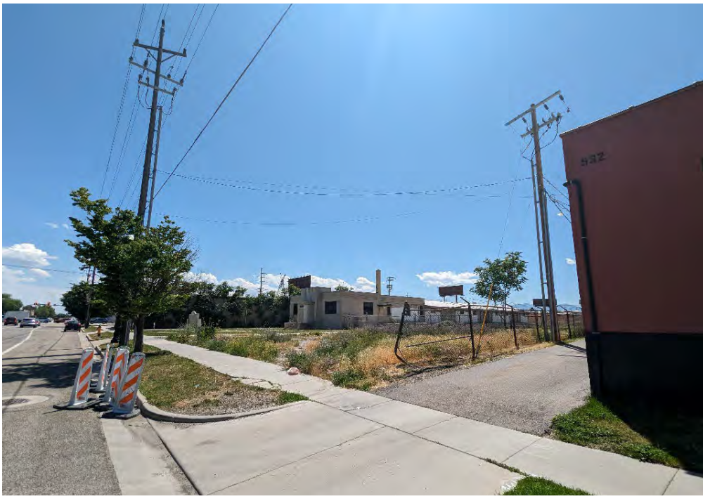
Proposed site of Building 2, northeast corner along 400 W
