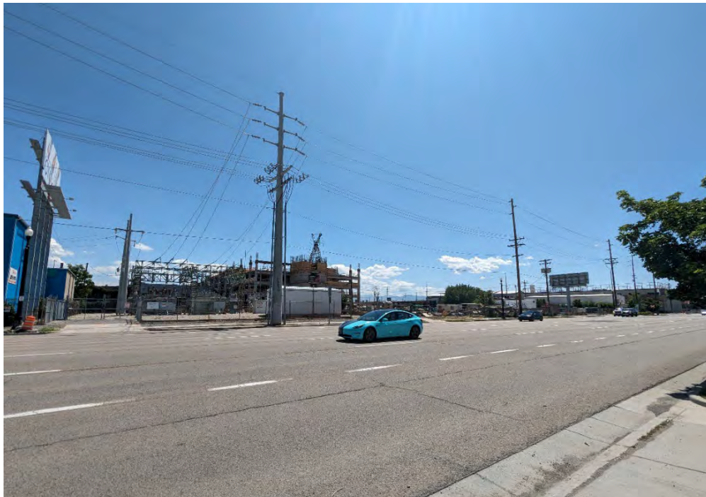
Neighboring property across 600 S
