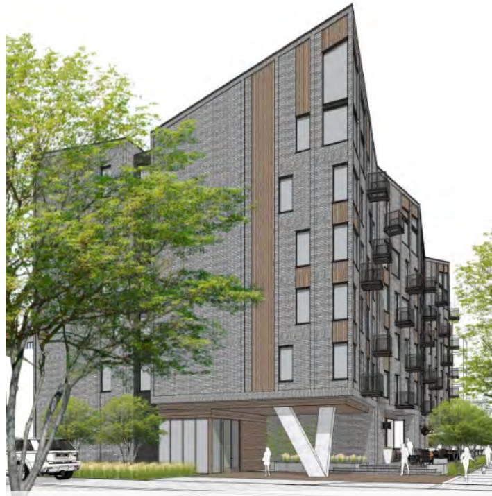
Building 1 – Southeast corner viewed from the midblock walkway.
