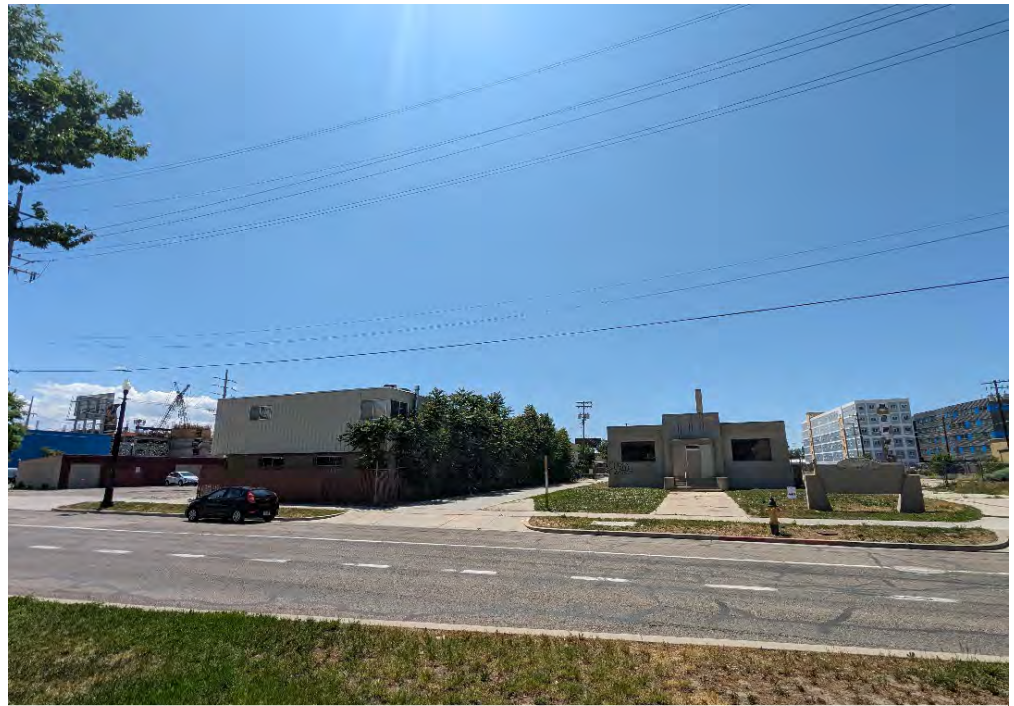
Proposed site of Building 2 along 400 W
