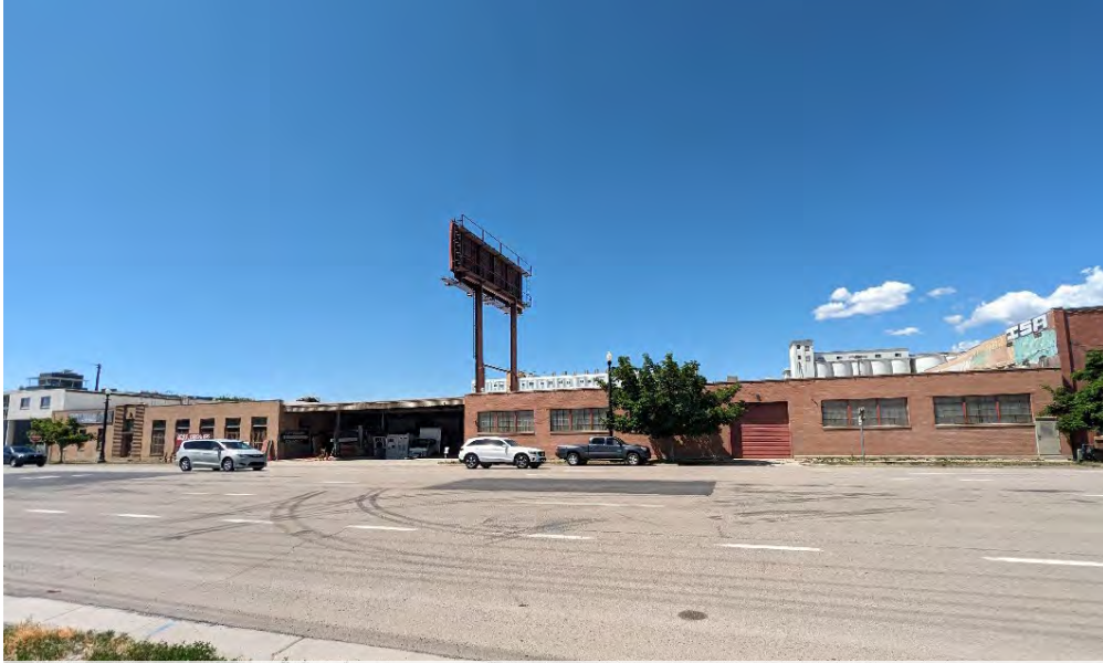
Miller Building along 600 S
