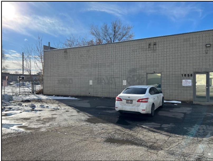
Closer view of building on south end of subject property
