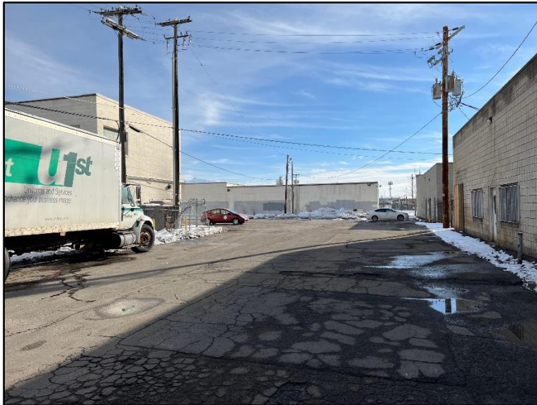
Current conditions of 1000 South Block of Washington Street
