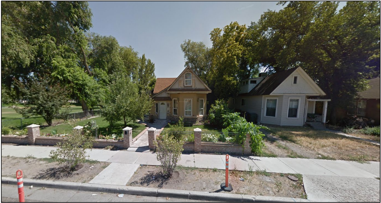
Previous single-family dwelling located at 135 W Goltz Ave
