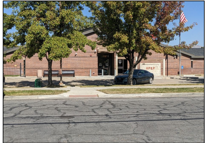
Commercial Building to the North (along Freemont)
