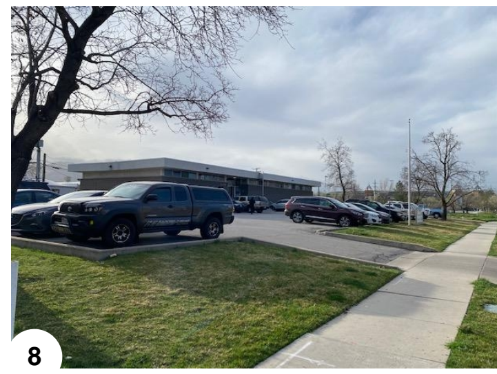
8 EXISTING BUILDING - NORTH
