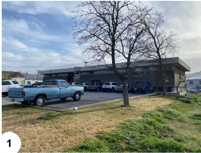
1 EXISTING BUILDING - SOUTH
