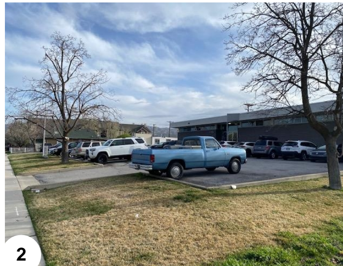
2 EXISTING BUILDING - SOUTH
