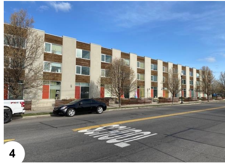
4 BUILDING ACROSS WEST TEMPLE
