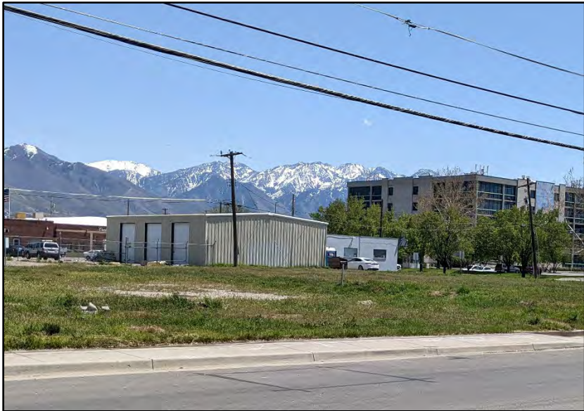
Vacant Land to the South and Nearby Development to the Southeast
