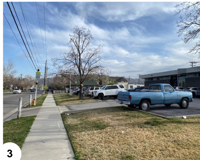
3 EXISTING BUILDING - SIDEWALK
