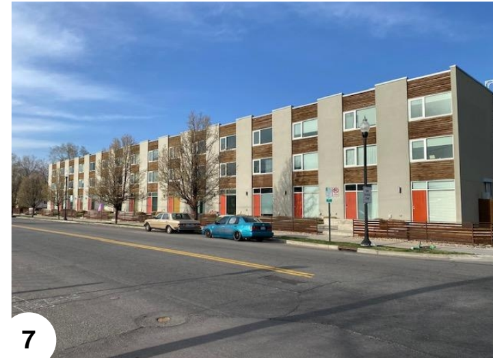
7 BUILDING ACROSS WEST TEMPLE
