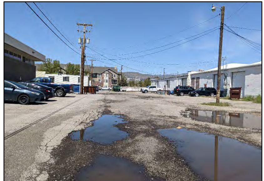
Alley to the Rear (East)
