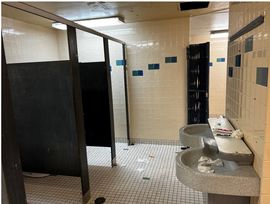
Figure 7: Current bathroom area
