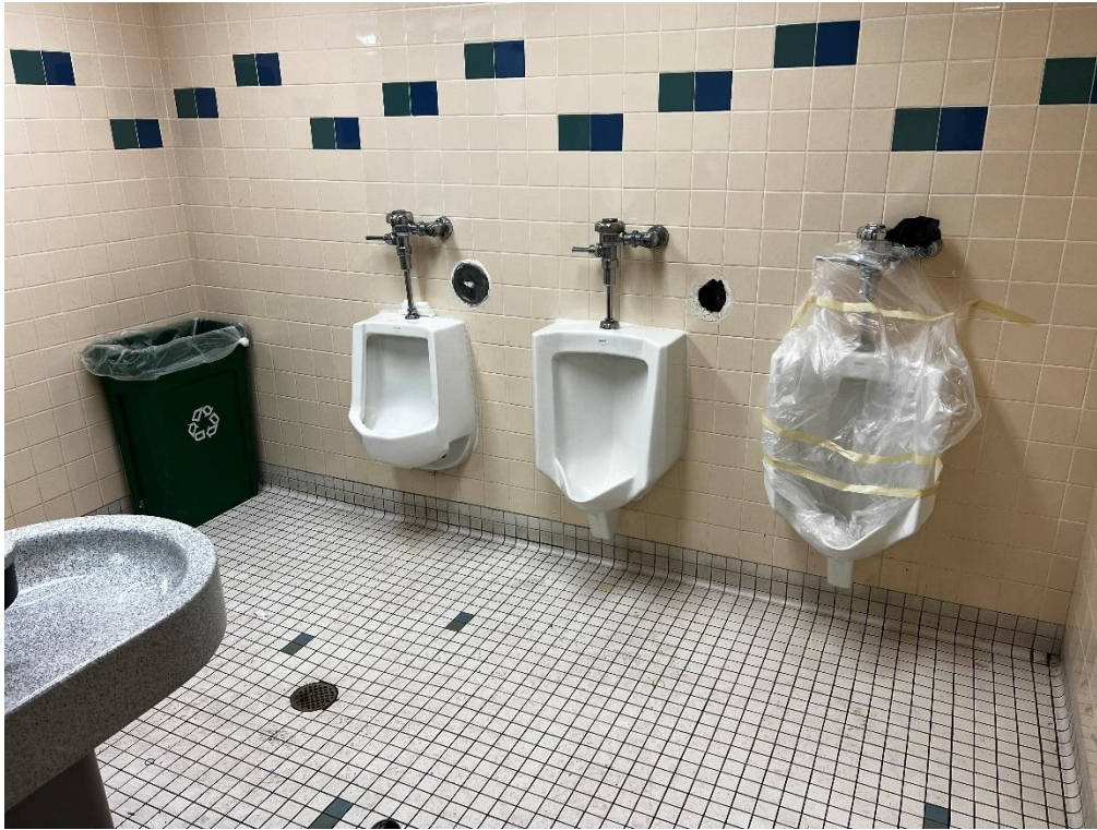
Figure 8: Men's restroom area
