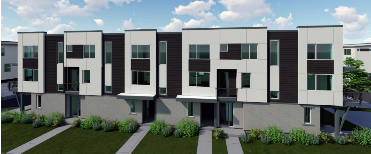
Central Building Fronting onto Redwood Road
