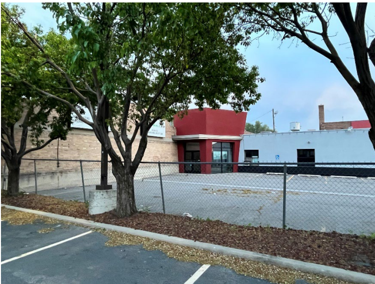
Business entrance at north side of 1435 South State Street
