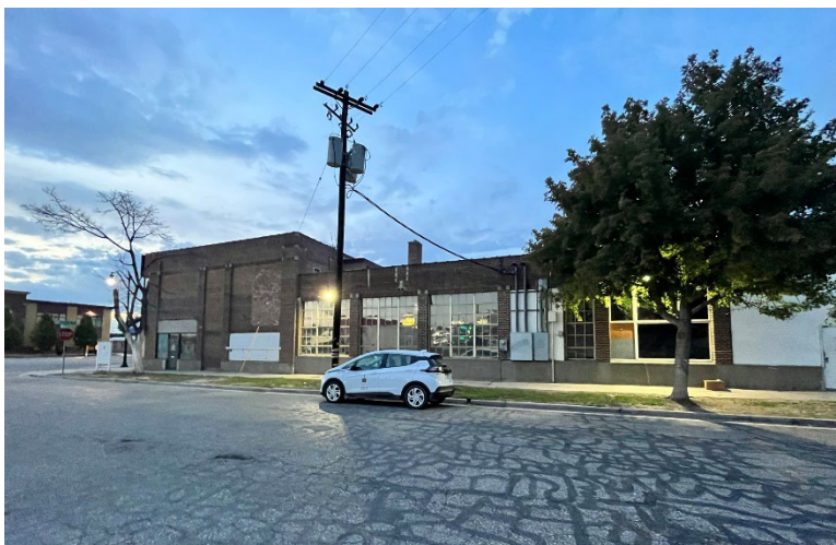
South Side of 1435 South State Street from Cleveland Avenue
