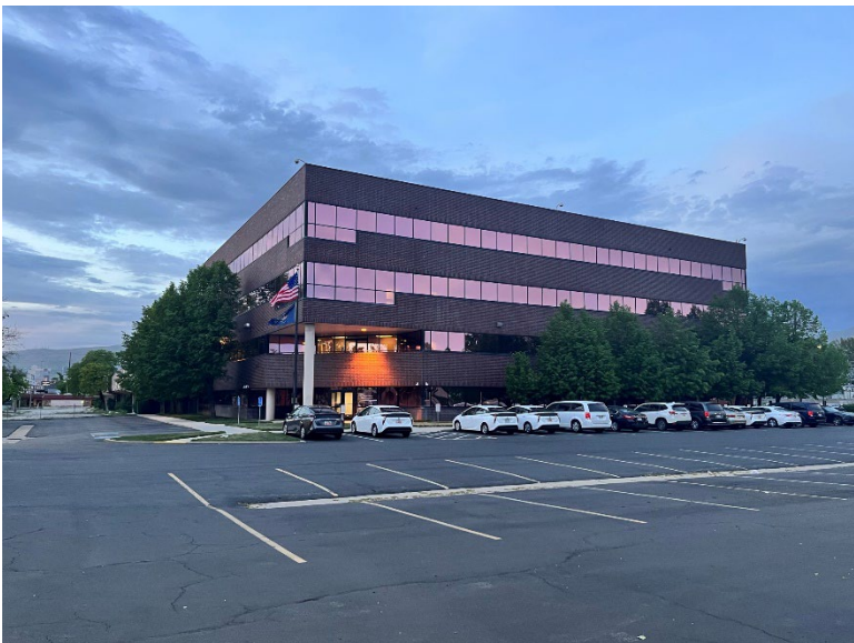
Utah Division of Child and Family Services Building at 1385 South State Street
