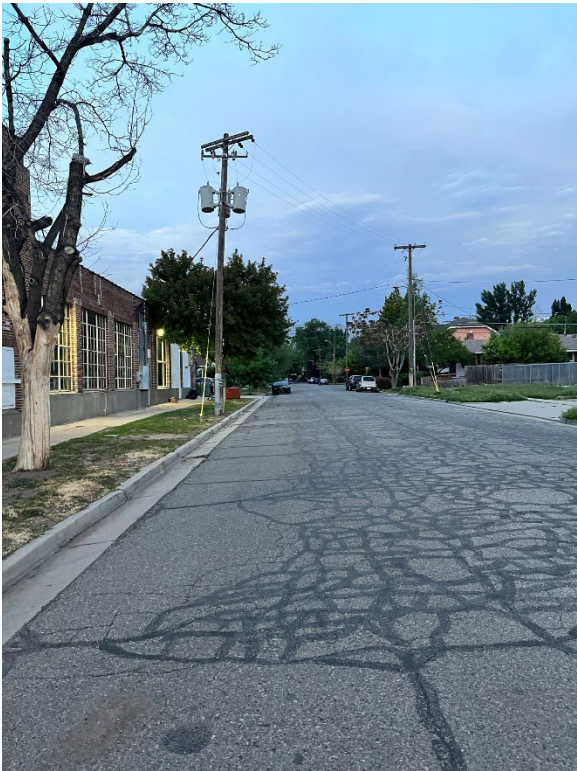
Cleveland Avenue and south wall of 1435 South State Street
