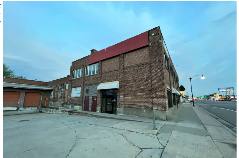
North Side of two-story brick commercial building on subject property
