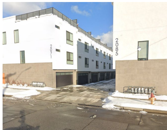
Figure 2: Example of a building encroaching on the sight distance triangle area
