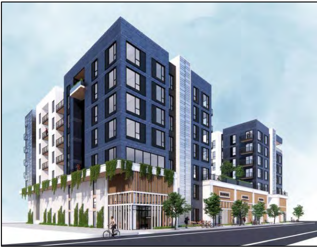
Northwest corner of the building - A 7 foot interior side yard setback has been provided for a future midblock connection.
