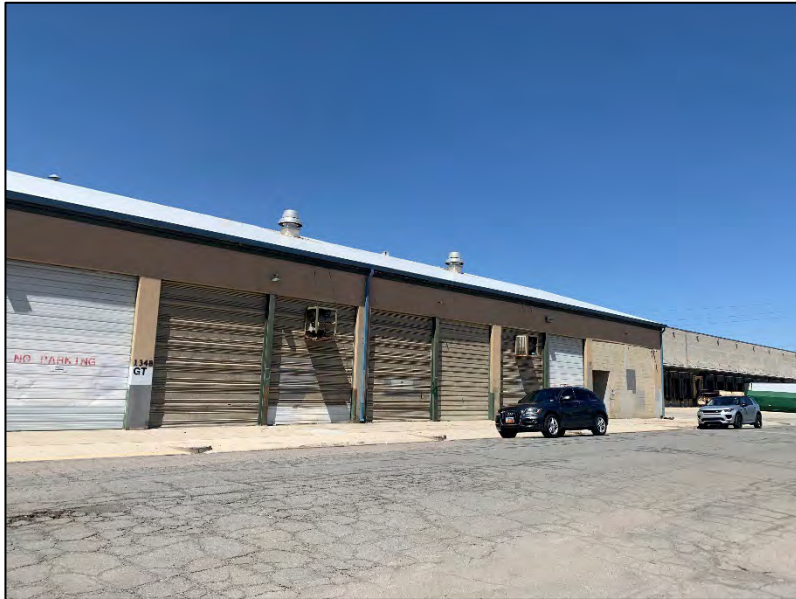
Property across Jefferson Street to the west
