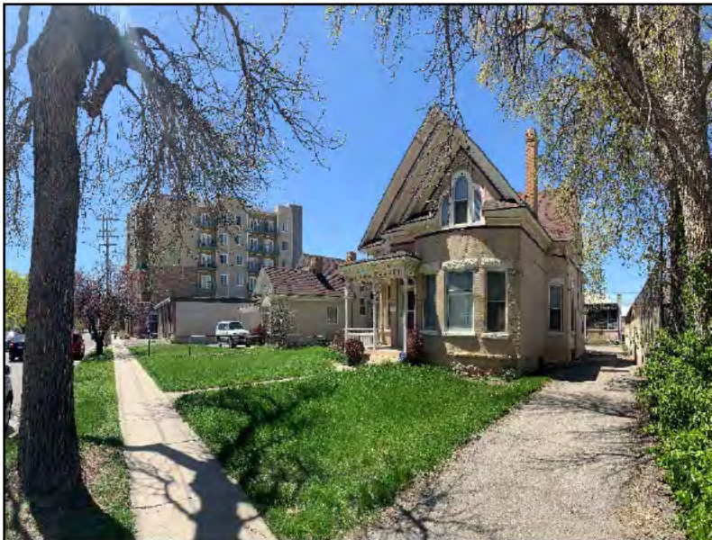
Properties to the east of the subject property on West Temple
