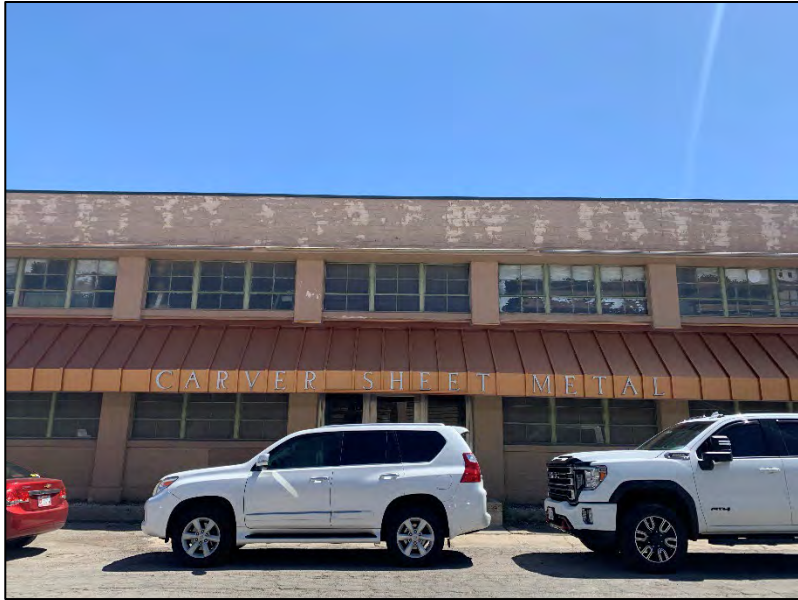
Front of the existing sheet metal building
