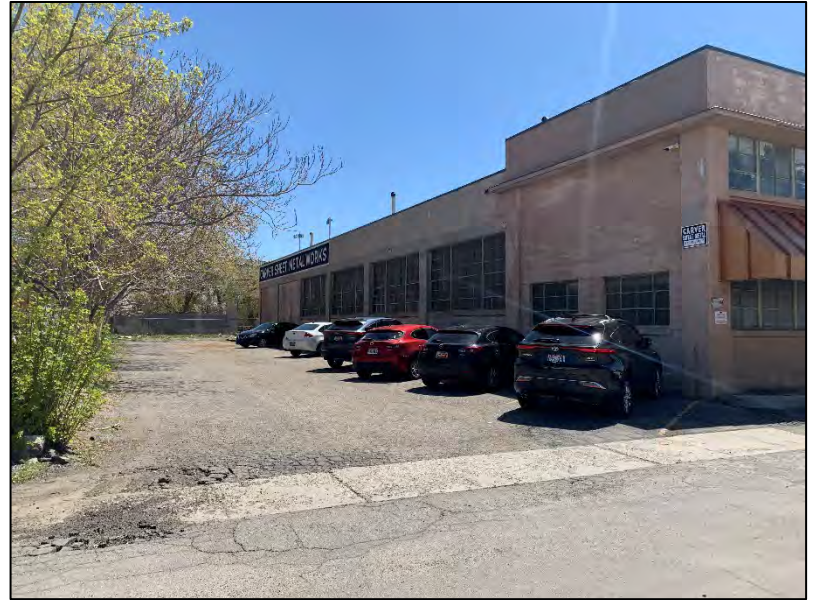
Northern side of the subject property
